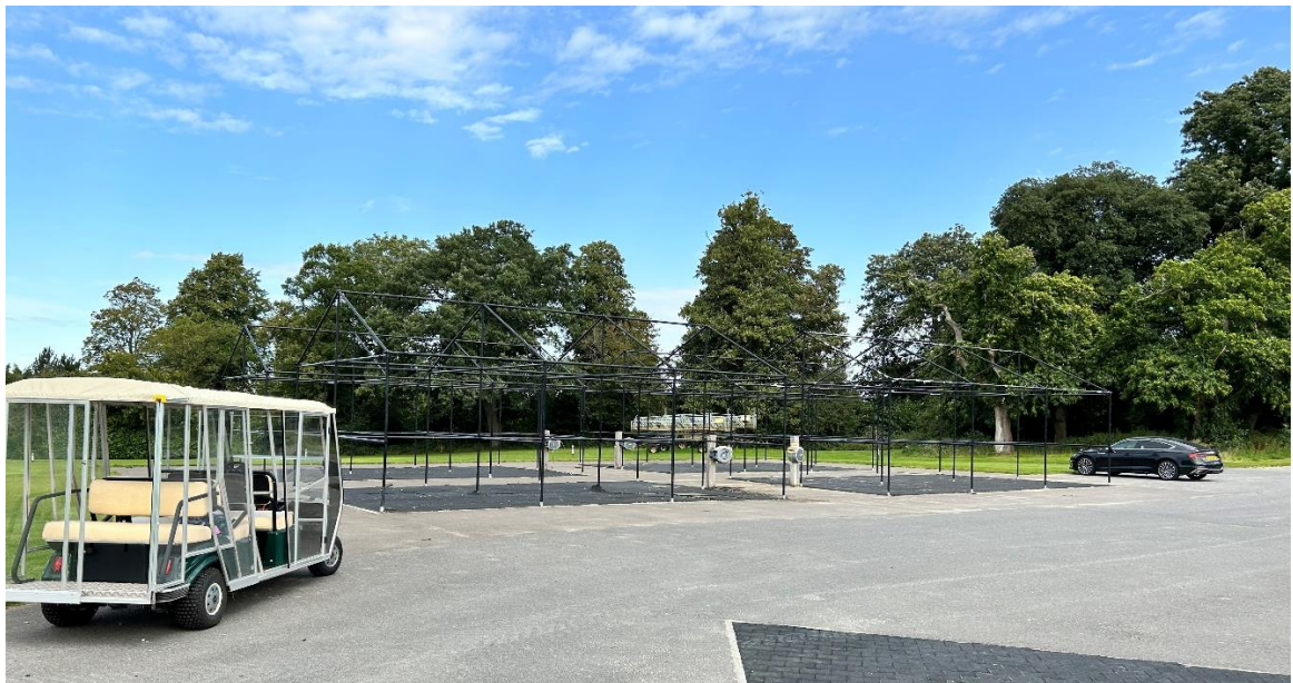
Fig. 1 – Pony lines marquee framework and additional area of hardstanding (Aug 2023)
