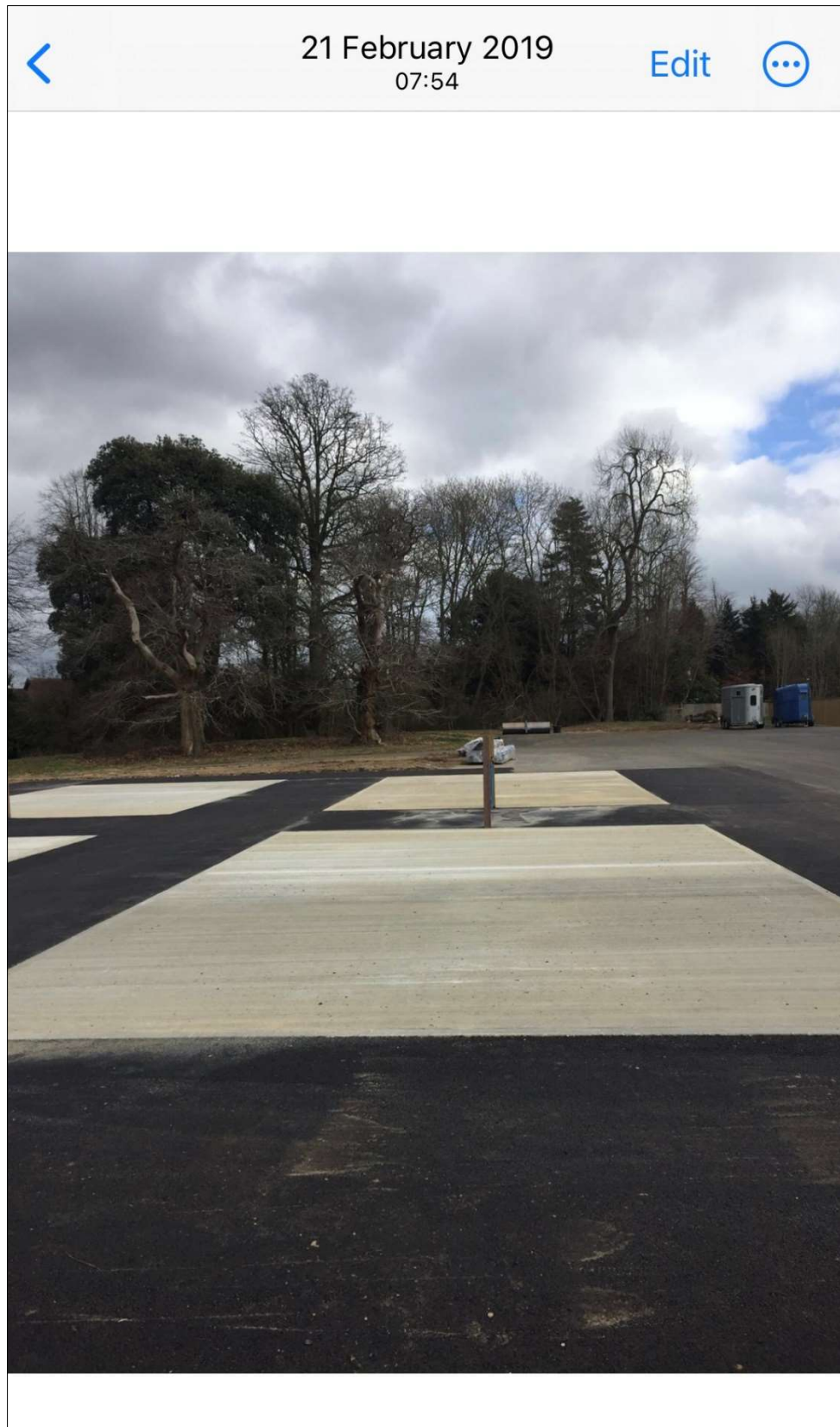
Photo. 1 – Concrete base of framework with extended asphalt hardstanding
