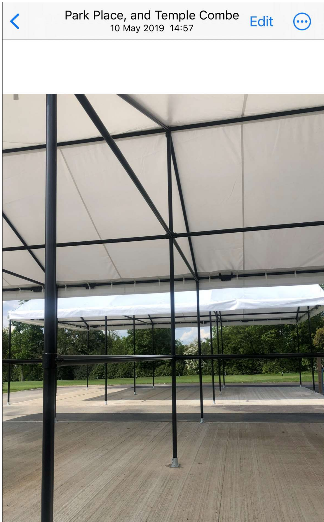
Photo. 3 – Frame with detachable roof covering
