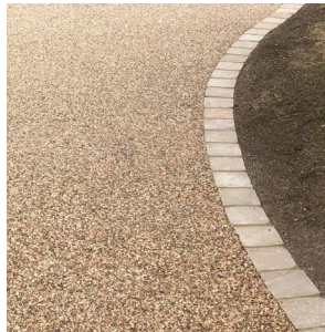
Setts edging to resin bound gravel
