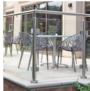
Balustrade to patio
