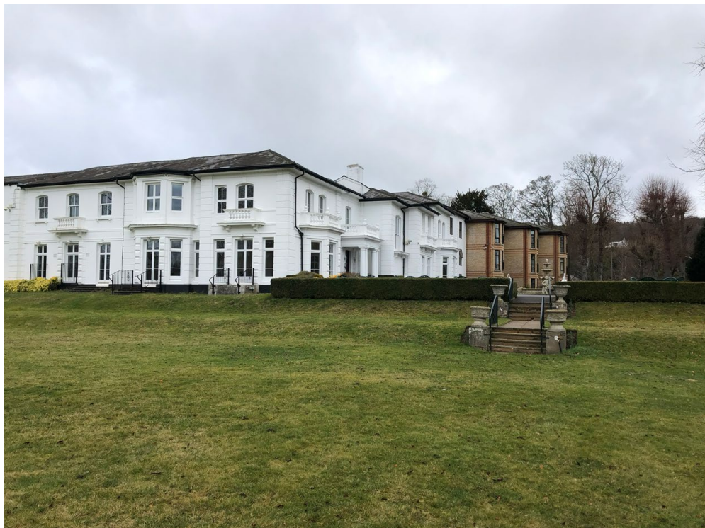
Figure 2.3: view from croquet lawn towards the Victorian part of Thamesfield House and the 1980s extension block
