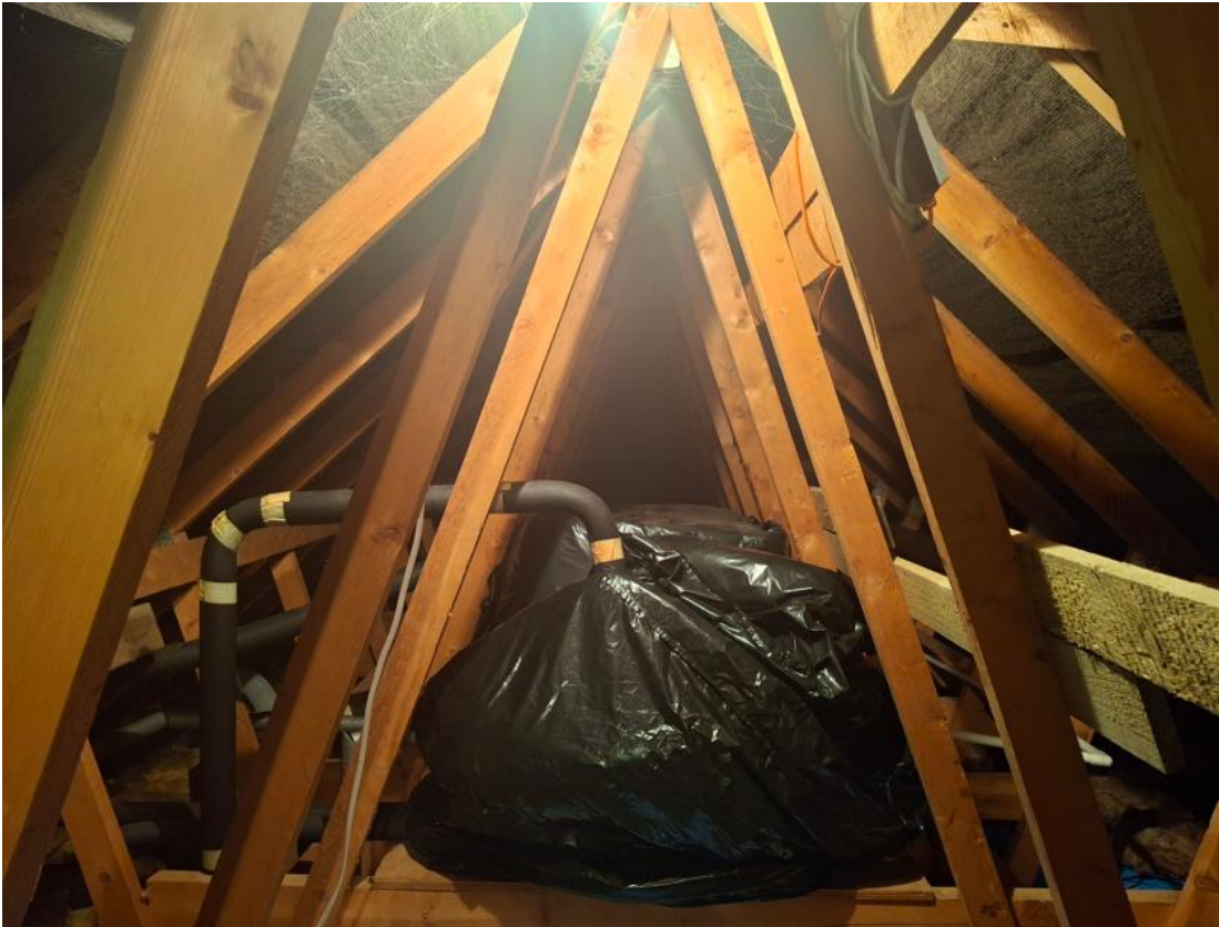
Figure 4: The loft void of B1
