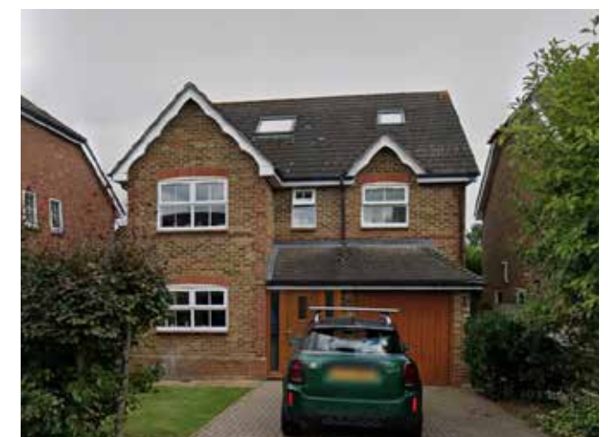
Figure 22: Photograph of Neighbouring Buildings Source: Google
