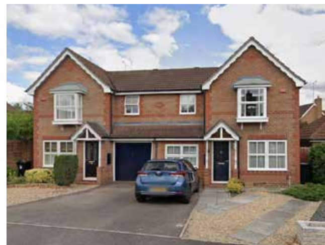
Figure 17: Photograph of Neighbouring Buildings Source: Google
