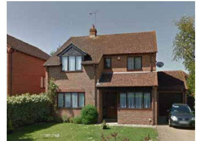
Figure 16: Photograph of Neighbouring Buildings Source: Google
