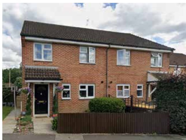
Figure 13: Photograph of Neighbouring Buildings Source: Google
