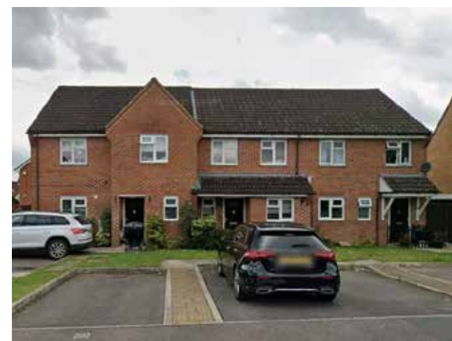
Figure 21: Photograph of Neighbouring Buildings Source: Google
