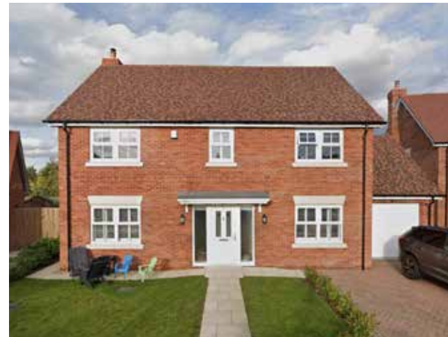
Figure 14: Photograph of Neighbouring Buildings Source: Google
