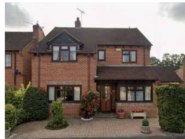
Figure 18: Photograph of Neighbouring Buildings Source: Google
