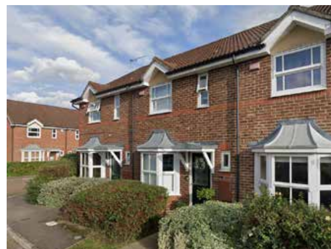
Figure 20: Photograph of Neighbouring Buildings Source: Google
