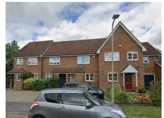
Figure 19: Photograph of Neighbouring Buildings Source: Google
