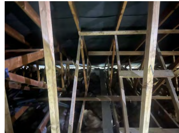
B1 internal void 1
