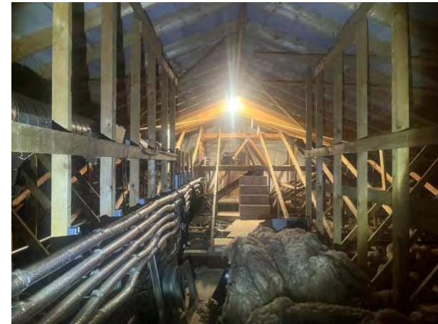
B1 internal void 1
