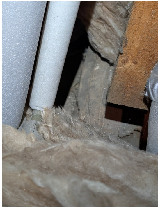
Photograph 6. Fractured beam underneath the water tank.
