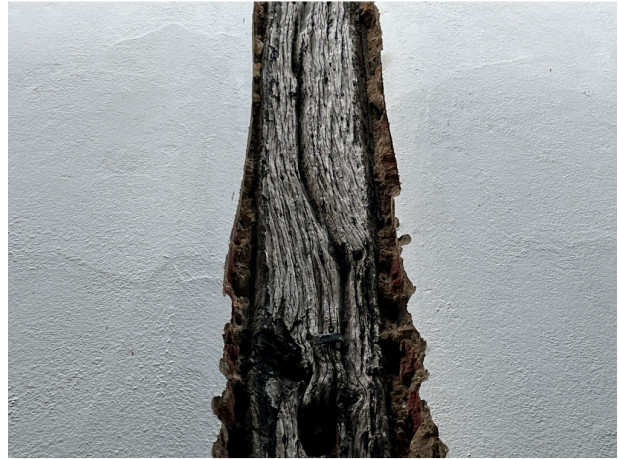
Photograph 8. Timbers to the exterior of the west facing gable end.
