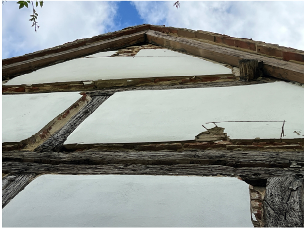
Photograph 7. West facing gable end.
