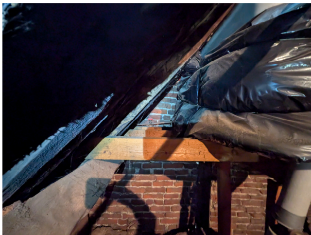
Photograph 1. View of west facing gable end.
