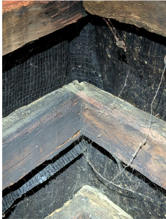
Photograph 4. Pegged rafters along the ridge.
