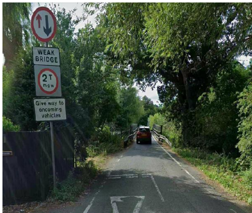
Weak bridge situated within Mill Lane to the north west of the site area
