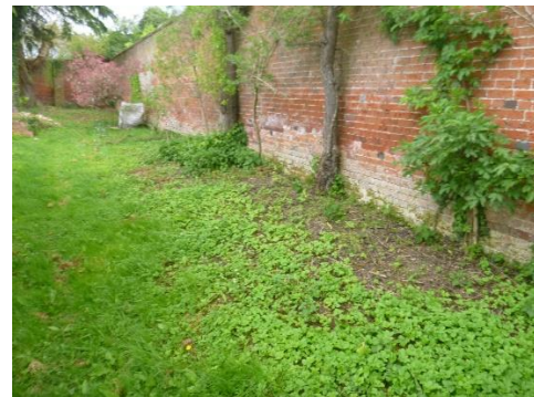
Photograph 12. Brick wall along the boundary.
