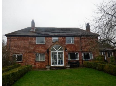
Photograph 2. House viewed from south.
