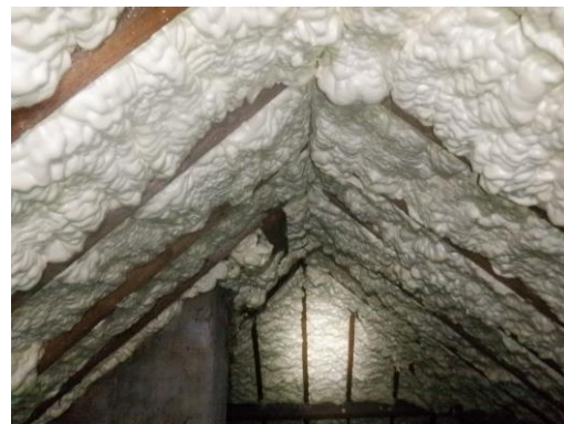
Photograph 14. Spray foam insulation covering entire roof.
