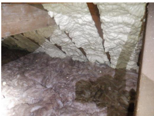
Photograph 15. Fibreglass insulation of floor throughout, eaves filled.
