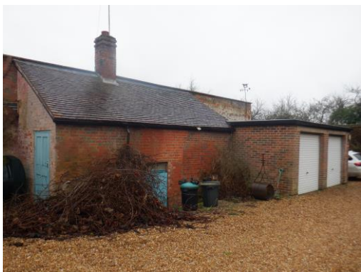
Photograph 3. View of single storey extension on the western elevation showing boiler room and garages viewed from north.
