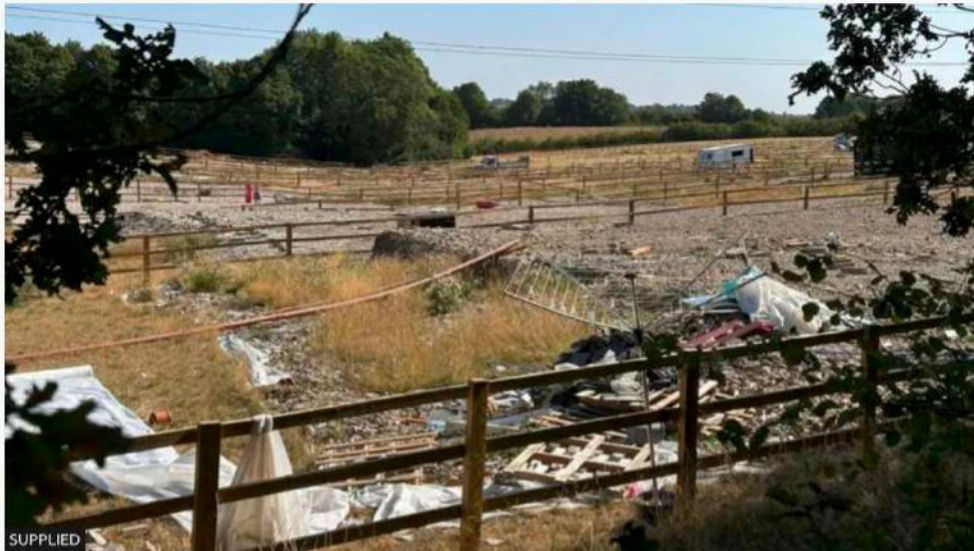
Pictured on 23 August, the site must be restored to its former state as grazing land
