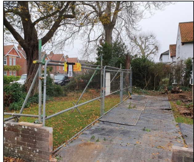
GP2: Tree protection barriers & trackmat ground protection
