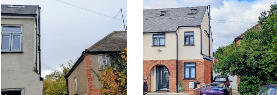
Fig 5:and 6 Lack of inset from boundary plus lack of subservience resulting in Dominance and overbearing of the side extension with respect to 26
