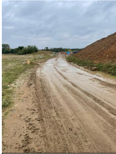
Road inside of site boundary, heading towards site compound.
