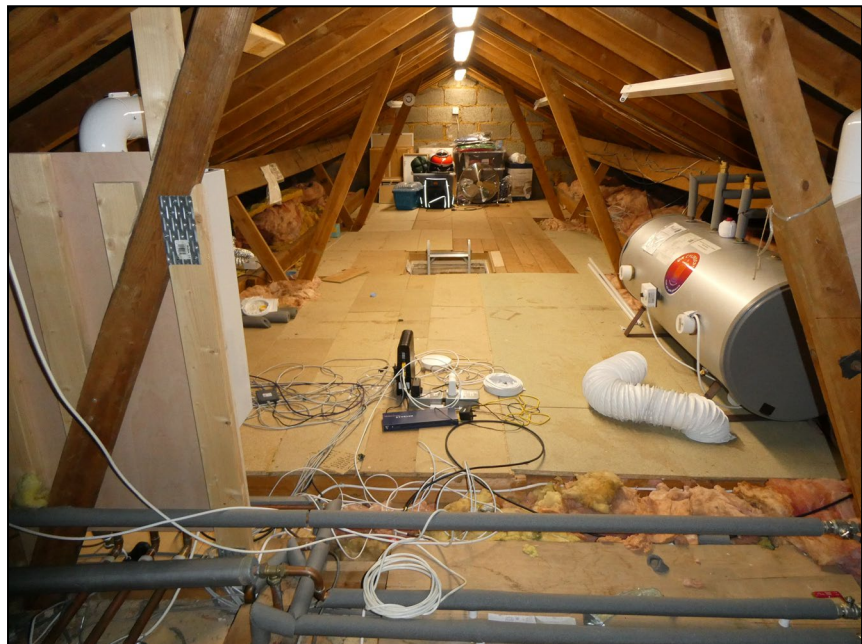
Figure 14. Example bitumen lining in main loft. 33 New Road, Ruscombe. 08.07.25
