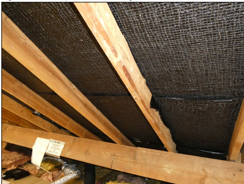
Figure 14. Example bitumen lining in main loft. 33 New Road, Ruscombe. 08.07.25
