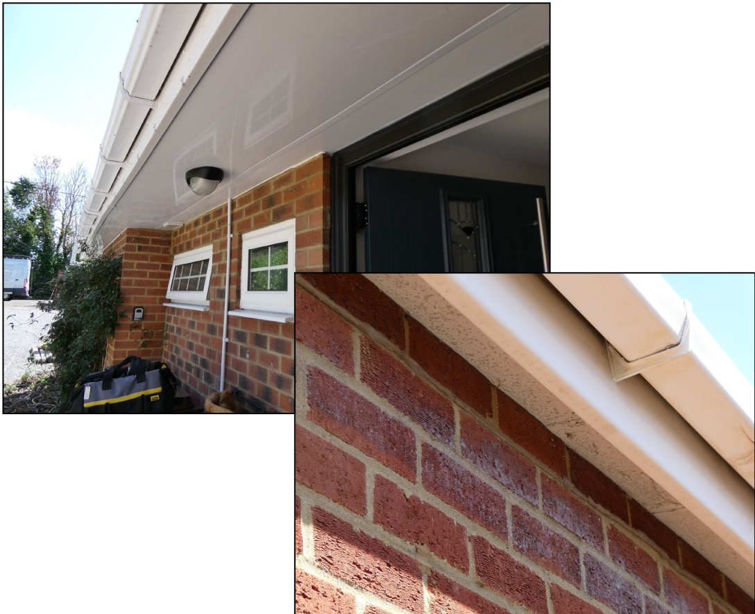
Figure 8. Example sealed uPVC soffits and fascias. 33 New Road, Ruscombe. 08.07.25
