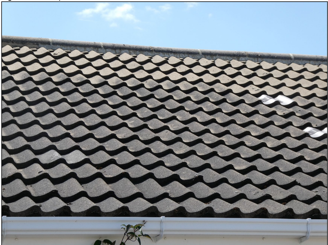
Figure 4. Example of roof tiles. 33 New Road, Ruscombe. 08.07.25
