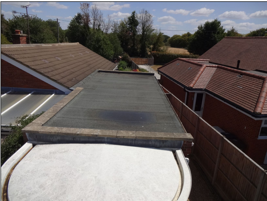
Figure 10. Bitumen covering flat roof extension. 33 New Road, Ruscombe. 08.07.25
