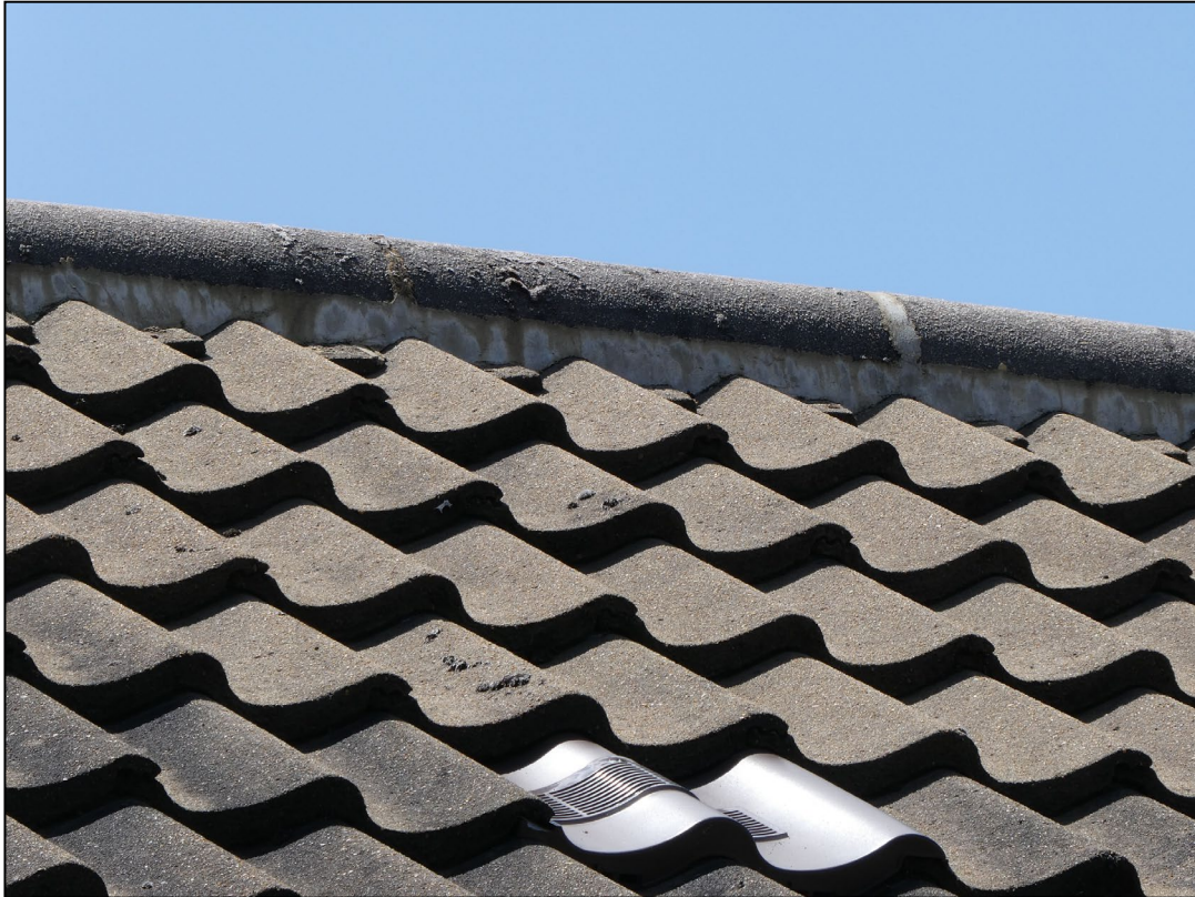
Figure 5. Example of ridge tiles. 33 New Road, Ruscombe. 08.07.25
