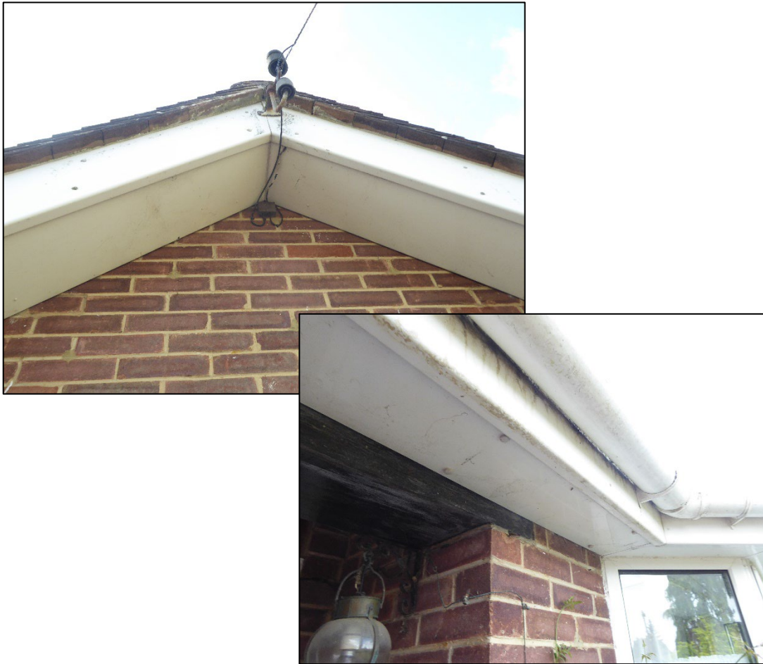
Figure 8. Example sealed soffits and fascias. 58 Redhatch Drive, Earley. 20.08.24
