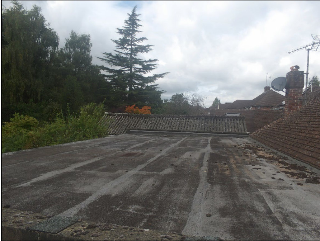
Figure 6. Example sealed bitumen felt on rear extension. 58 Redhatch Drive, Earley. 20.08.24
