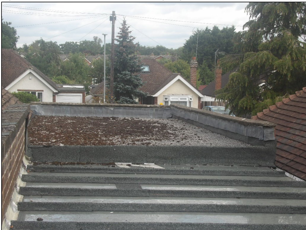
Figure 7. Example sealed bitumen felt on garage. 58 Redhatch Drive, Earley. 20.08.24
