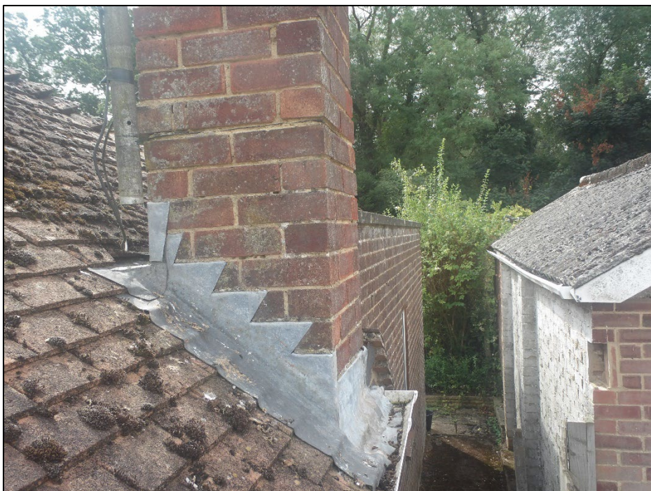
Figure 9. Example lead flashing on chimney stack. 58 Redhatch Drive, Earley. 20.08.24
