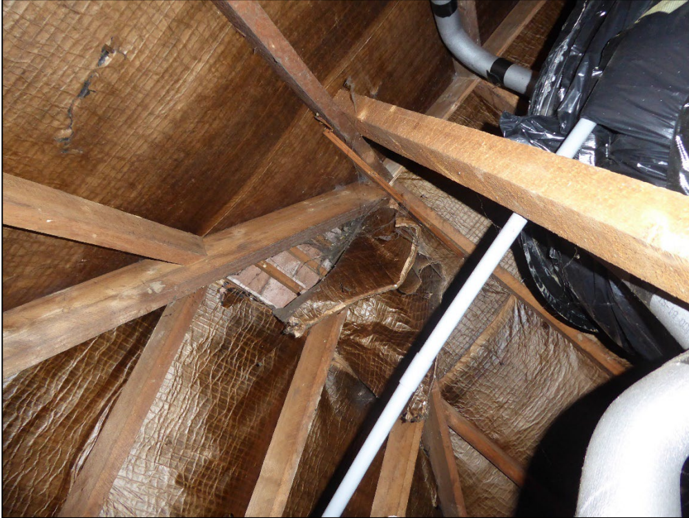
Figure 11. Example torn tar paper lining to roof tiles. 58 Redhatch Drive, Earley. 20.08.24
