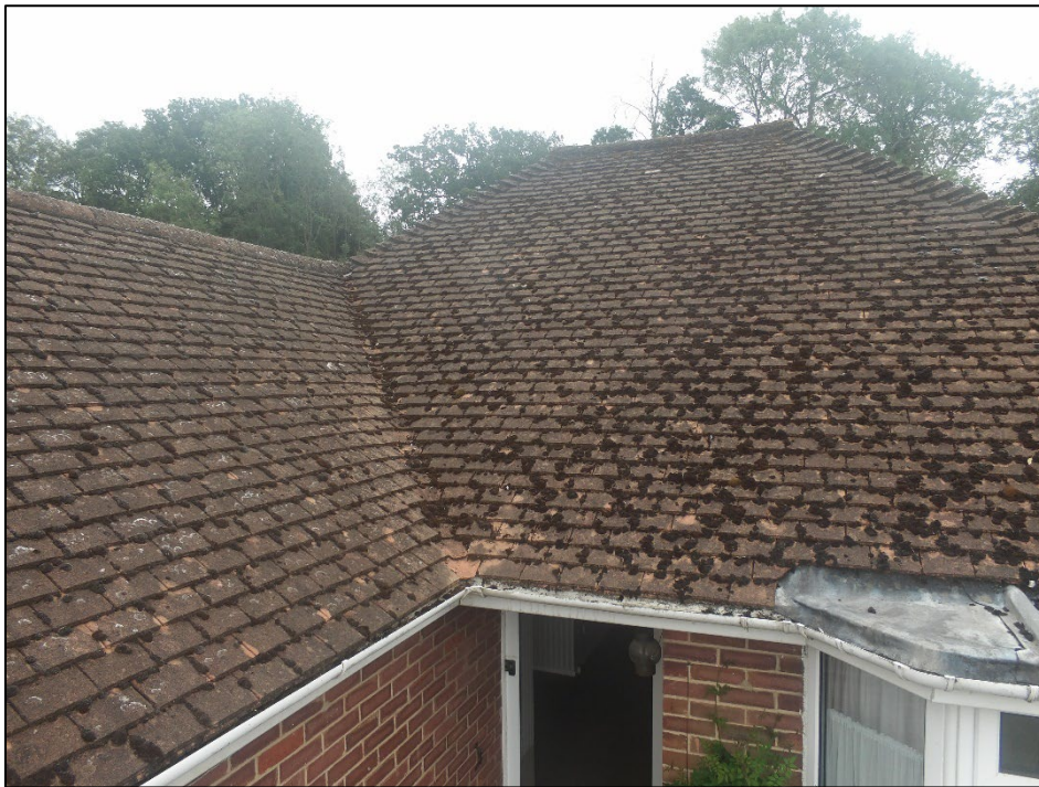
Figure 5. Example of sealed hip tiles. 58 Redhatch Drive, Earley. 20.08.24
