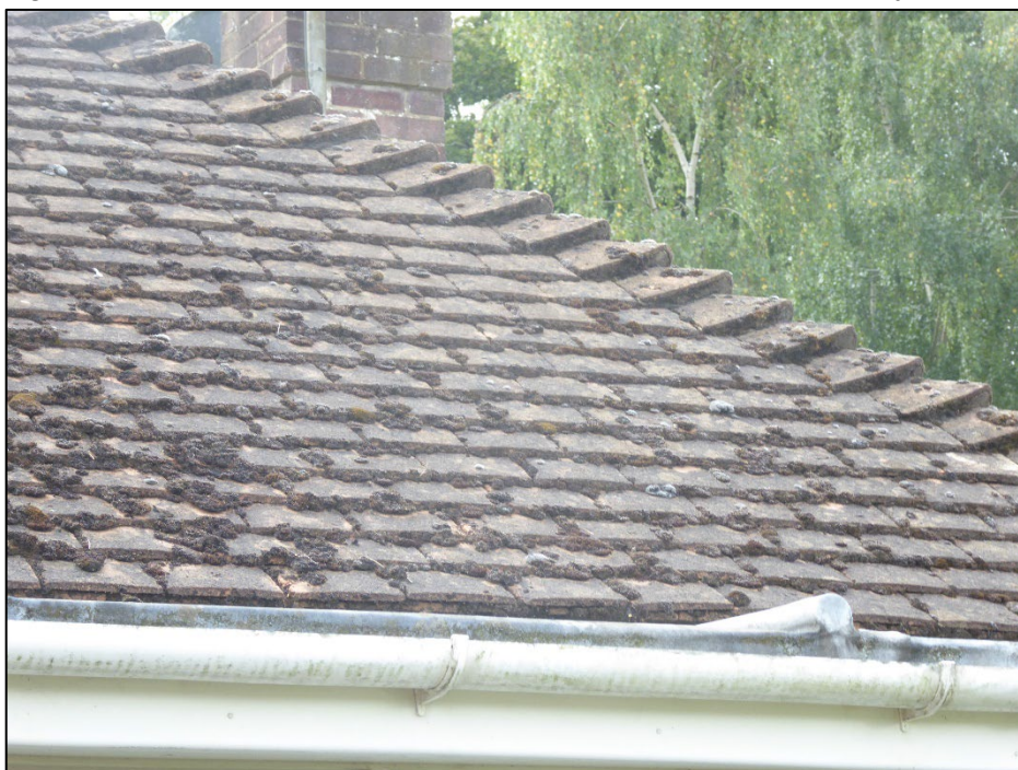
Figure 5. Example of sealed hip tiles. 58 Redhatch Drive, Earley. 20.08.24
