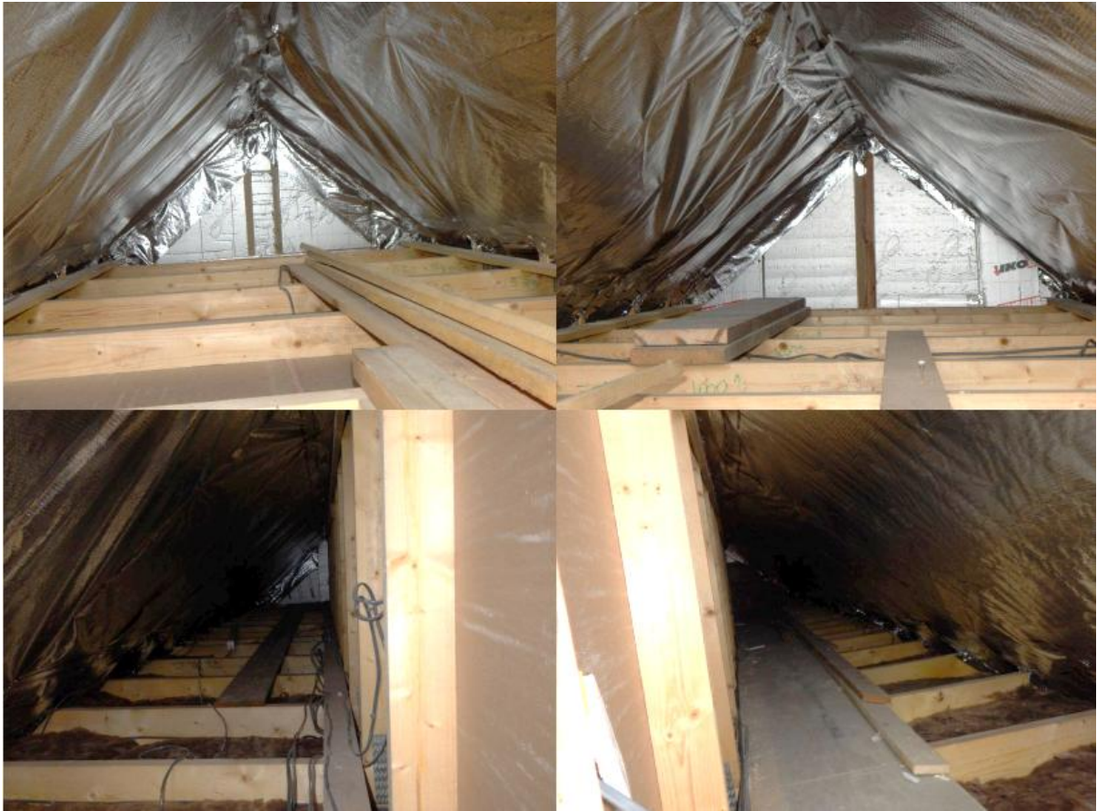
Image 7 – Internal views from within the accessible roof void spaces of the property
