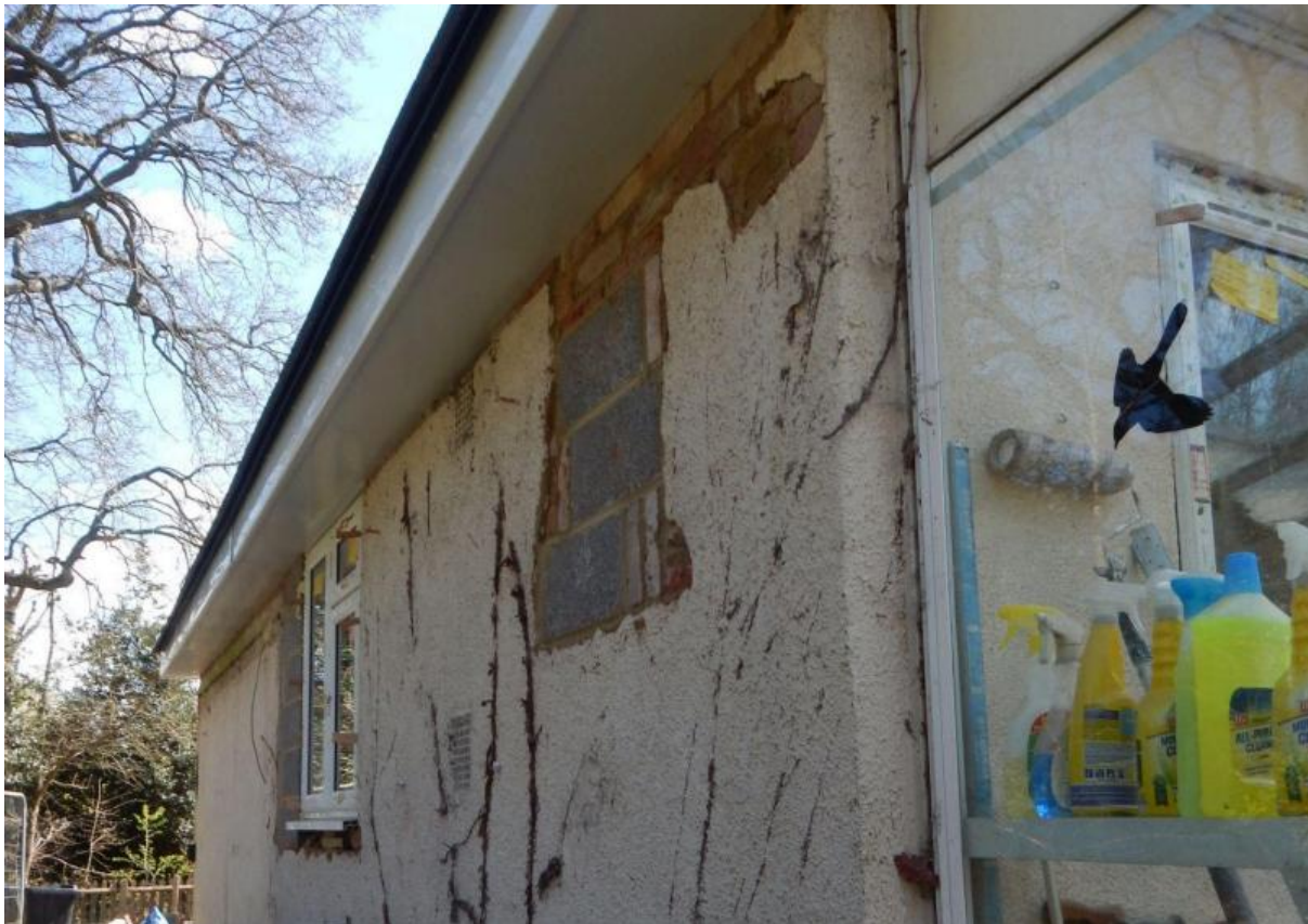
Image 4 – North facing elevation of the property
