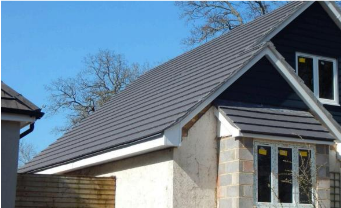
Image 3 – South facing elevation of the property
