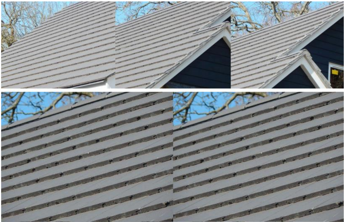
Image 5 – Example images of the tiled roof coverings to demonstrate condition throughout
