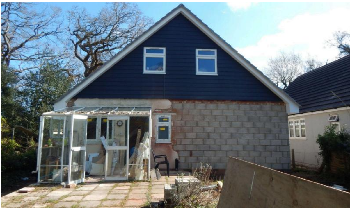
Image 2 – West facing elevation of the property
