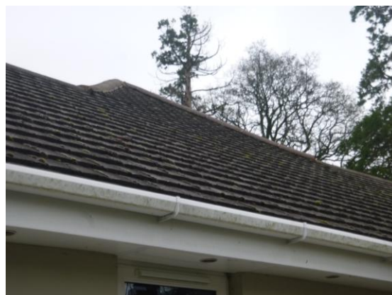
Photograph 4. Ridge and hip tiles fully mortared (southern elevation).
