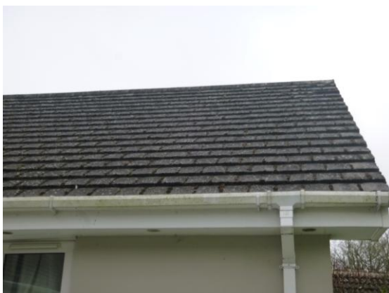
Photograph 3. Flat plain tiles (northern/rear elevation).
