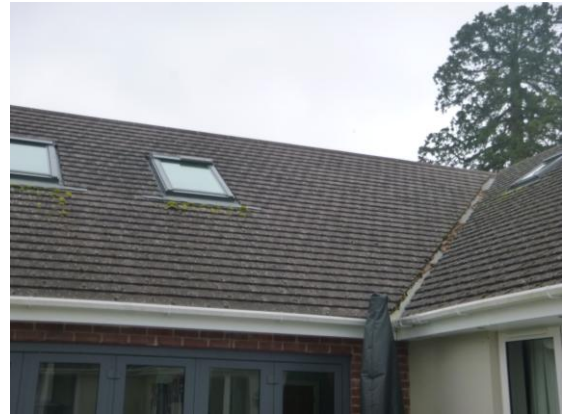
Photograph 7. Tight corrugated sheeting under rooflights (rear elevation).
