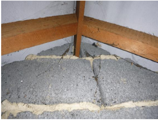
Photograph 14. Rear gable end.
