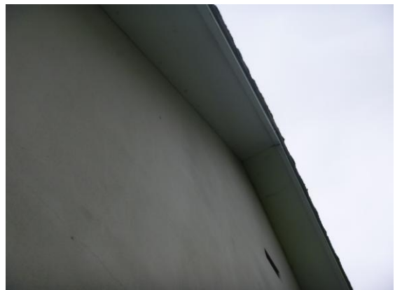
Photograph 9. uPVC soffit flush at southern gables (rear elevation).
