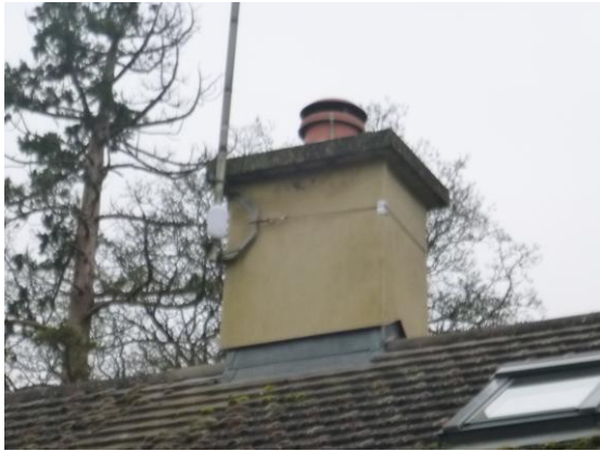
Photograph 6. Tight lead flashing around chimney (rear elevation).
