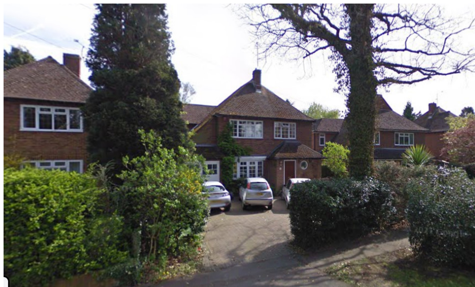
Asymmetrical pitched roofs and dropped eaves
