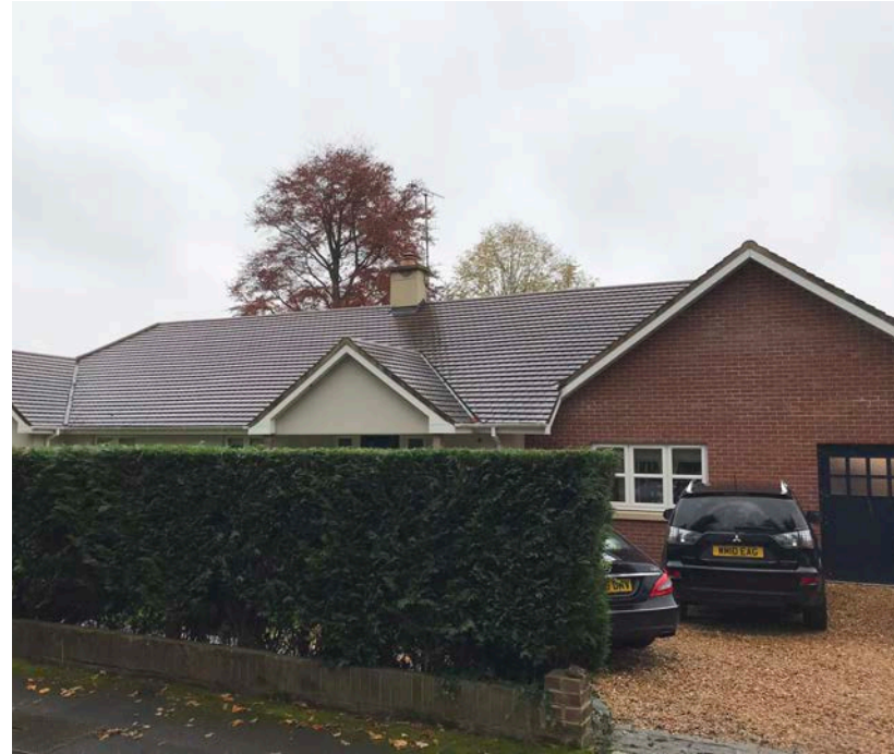
Above Left - View showing boundary hedge to the front garden of the property fronting Frog Hall Drive
