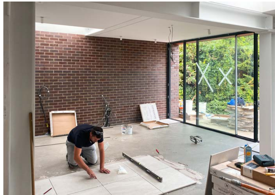
Work in progress, Lambeth, London
