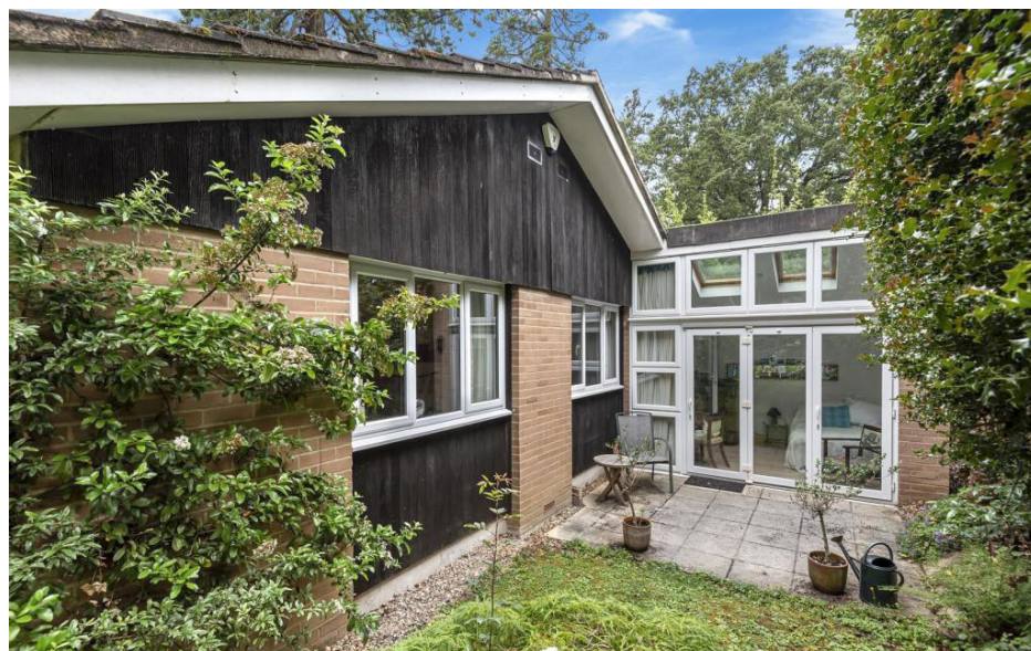
Single storey - 48 Frog Hall Drive
