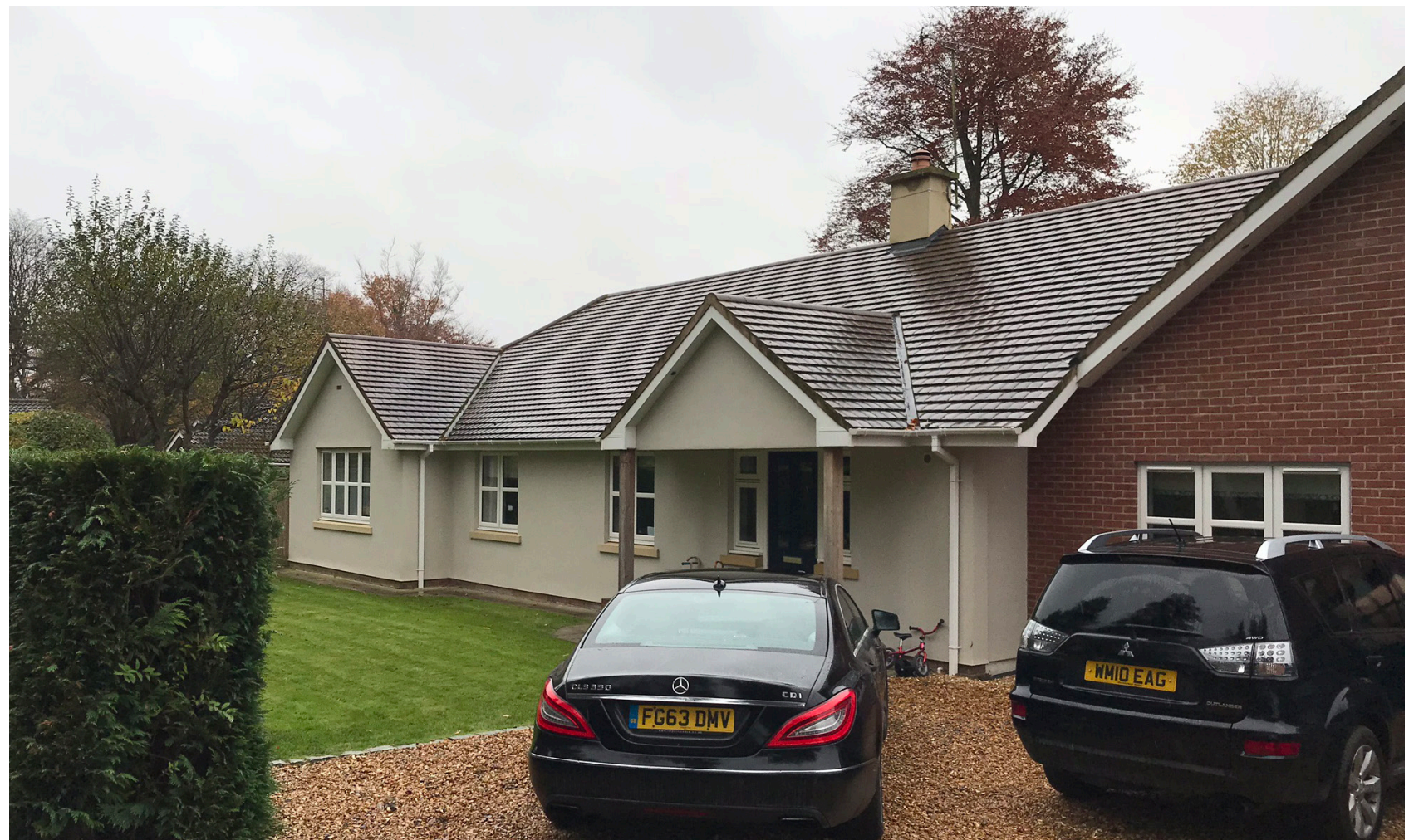
Below - Front elevation and driveway
