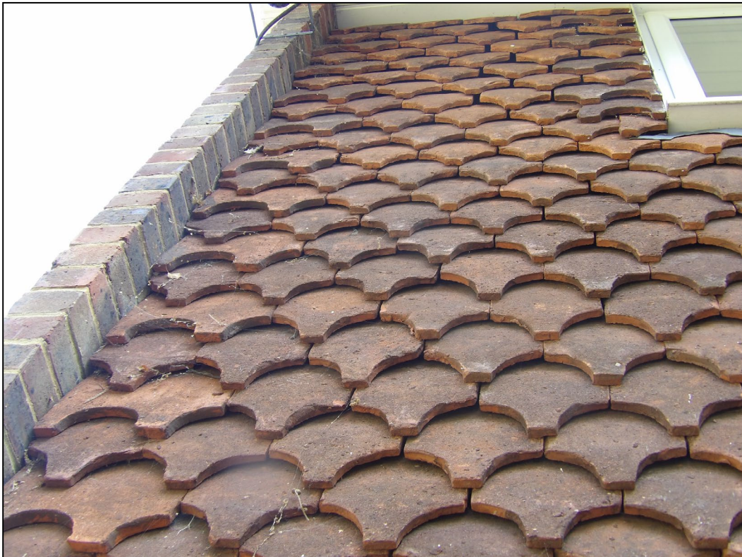
Figure 8. Example gaps in hanging tiles. 7 Greenside, Crowthorne. 12.08.25
