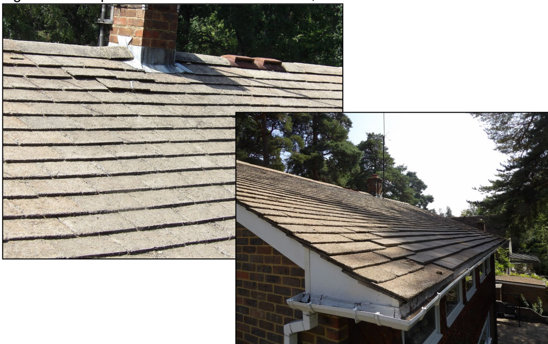
Figure 4. Example raised roof tiles. 7 Greenside, Crowthorne. 12.08.25
