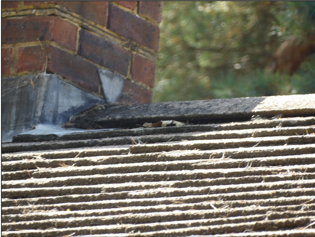
Figure 5. Example gaps in ridge tiles. 7 Greenside, Crowthorne. 12.08.25
