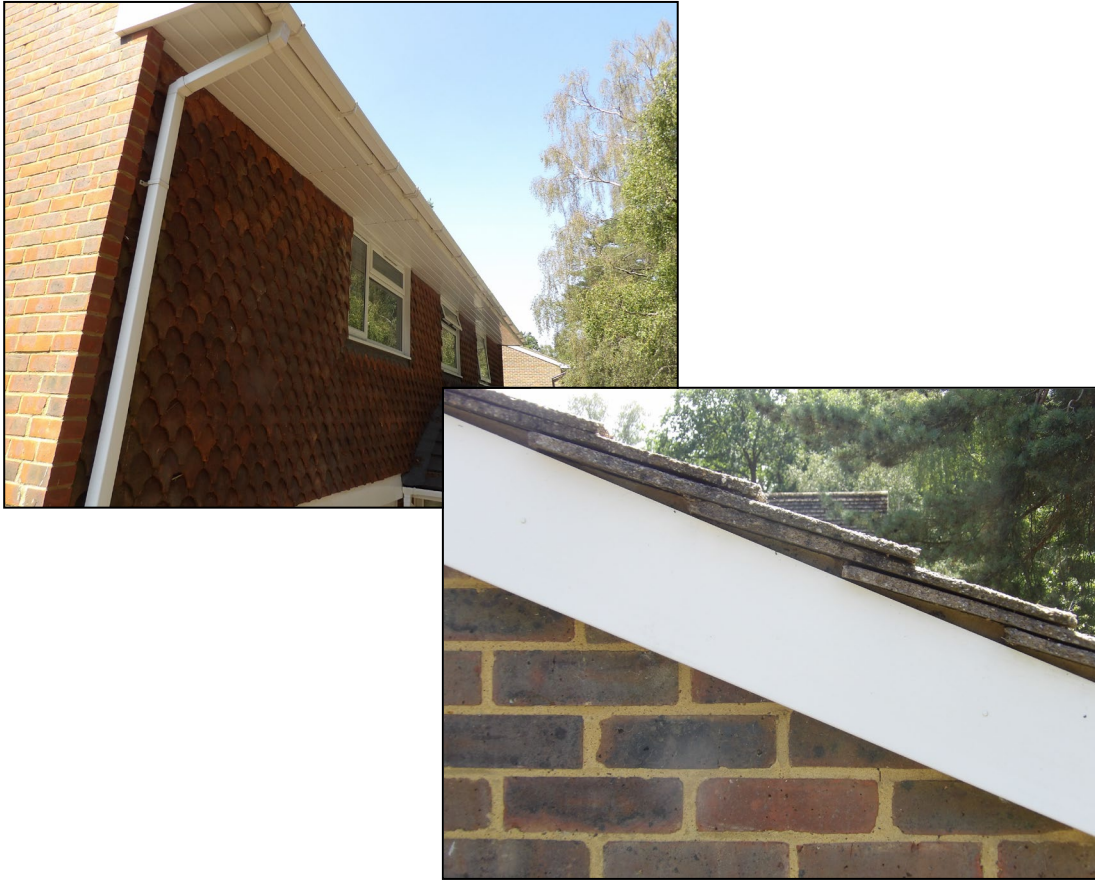
Figure 8. Example gaps in hanging tiles. 7 Greenside, Crowthorne. 12.08.25
