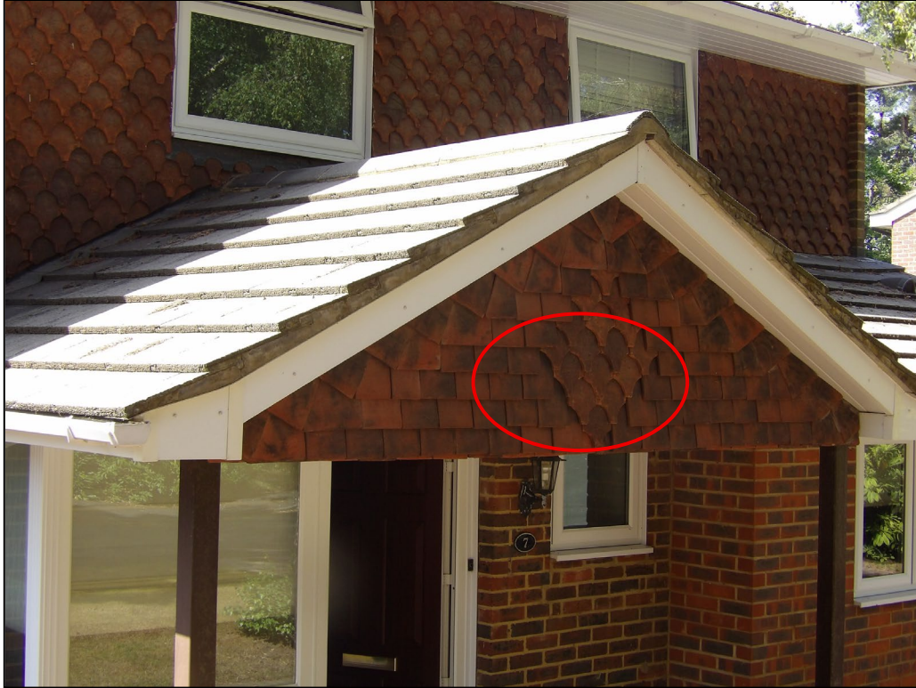
Figure 9. Front porch with moved hanging tiles with gaps. 7 Greenside, Crowthorne. 12.08.25
