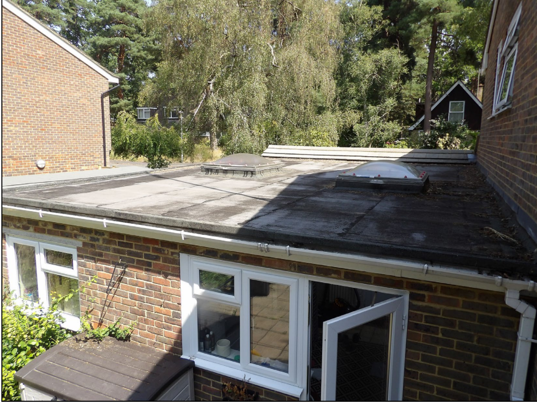
Figure 11. Example sealed bitumen felt on car port/garage. 7 Greenside, Crowthorne. 12.08.25
