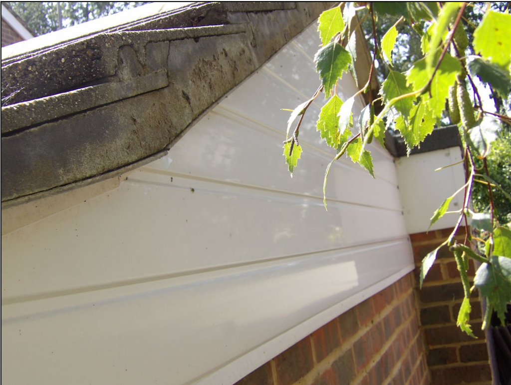
Figure 12. Example sealed verges and fascias on car port/garage. 7 Greenside, Crowthorne. 12.08.25
