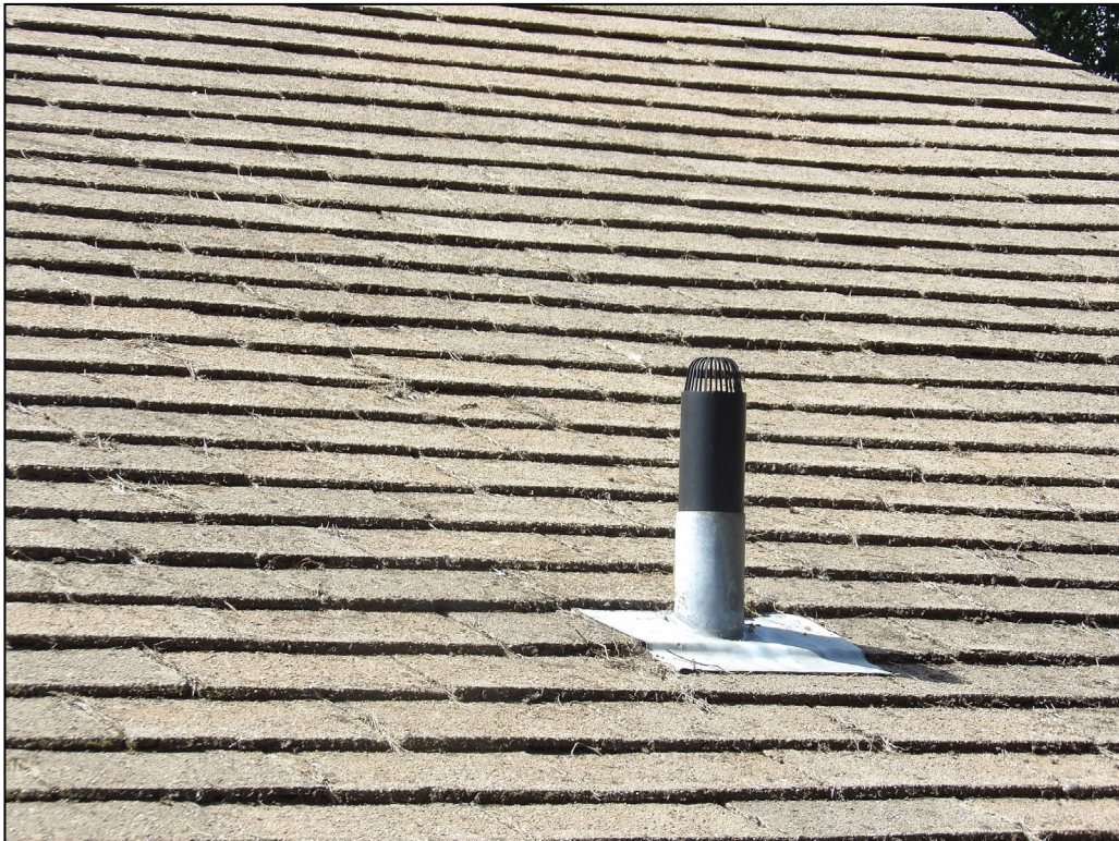
Figure 6. Example sealed lead flashing. 7 Greenside, Crowthorne. 12.08.25
