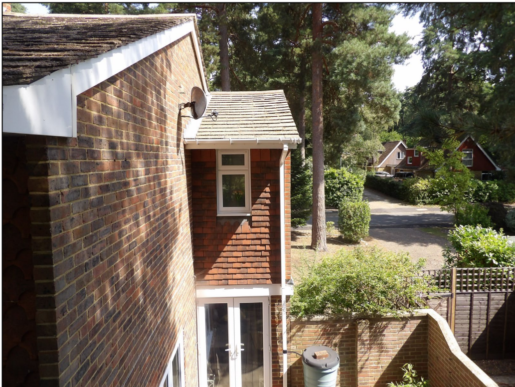
Figure 10. Subservient side section of property and hanging tiles. 7 Greenside, Crowthorne. 12.08.25
