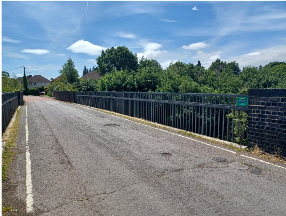
Photograph taken 21/05/26 showing brick parapet with metal railings.
