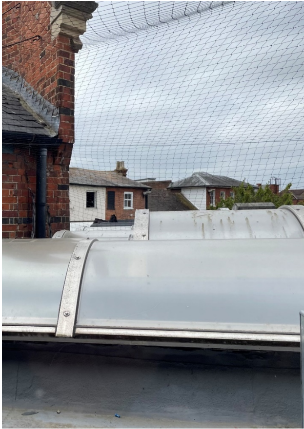
Courtyard roof raised Perspex lights. Top line of the parapet upstand around courtyard circled in blue. The 2no. Perspex rooflights (one covered in black cloth) would be where ASHP to be situated.
