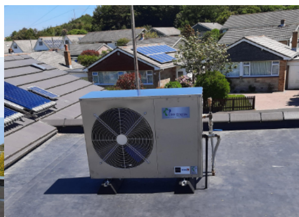
An example of a cantilevered free-standing railing. An example of anti-vibration mounts for a ASHP unit,
