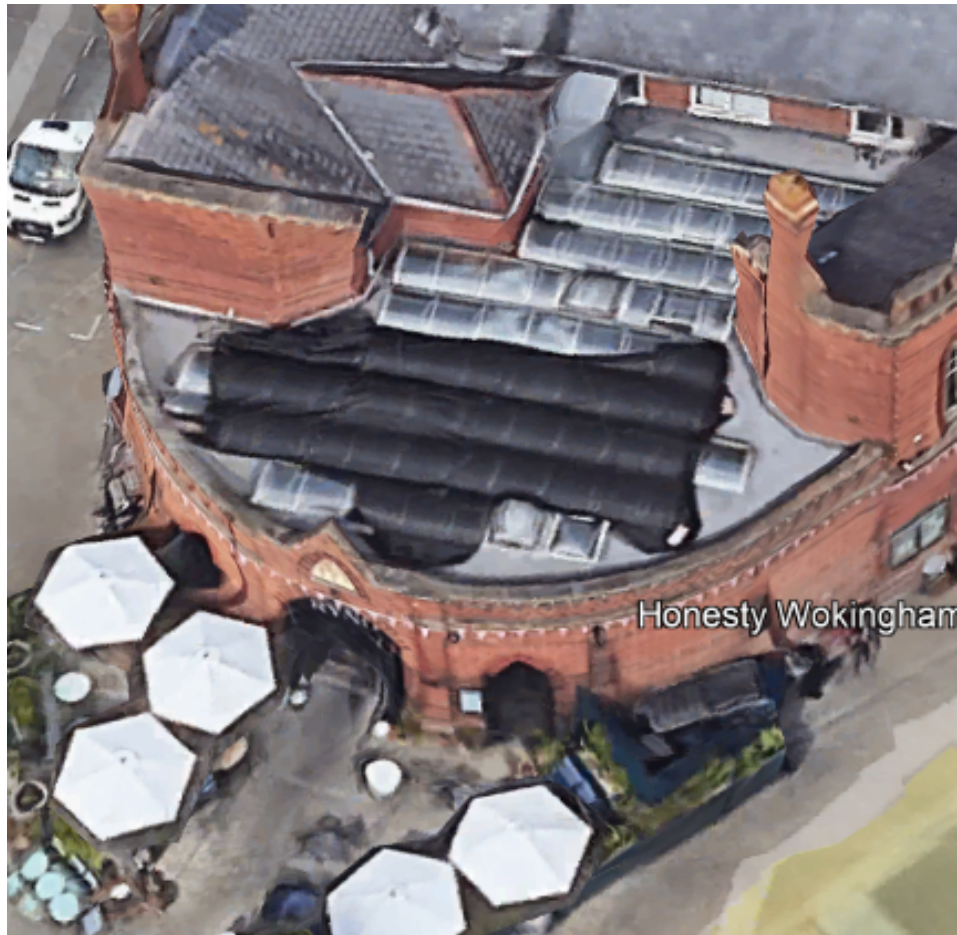
Aerial photograph of courtyard roof,
