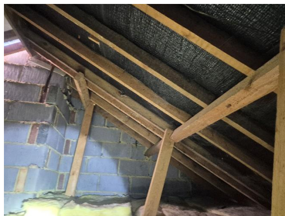
Photograph 8: Loft void of B1.
