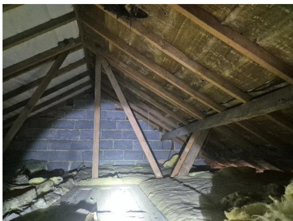
Photograph 7: Loft void of B1.
