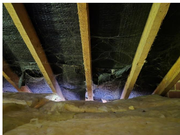
Photograph 10: Light ingress at the northern side of the loft void of B1.
