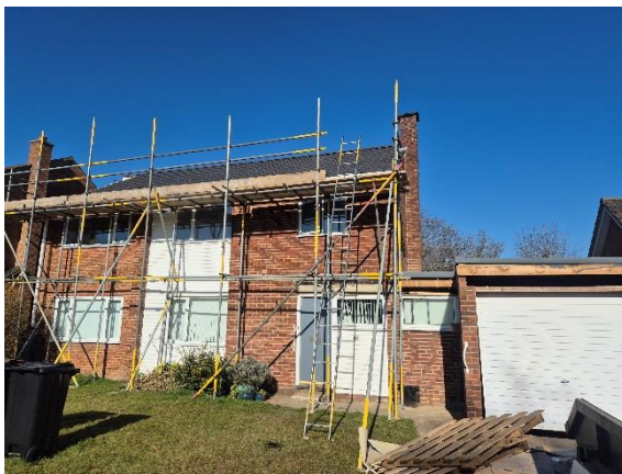
Photograph 1: Southern elevation of B1.
