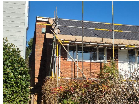
Photograph 2: Western elevation of B1.
