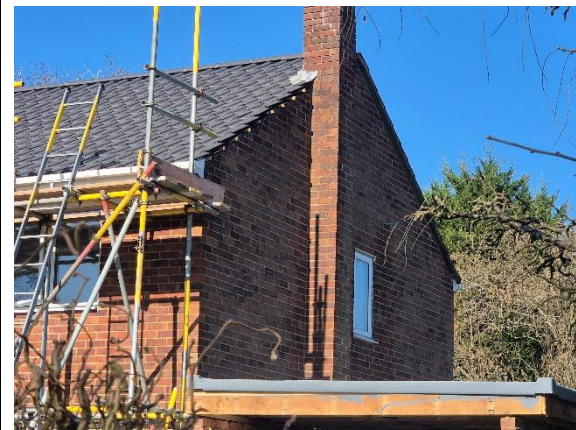
Photograph 4: Eastern elevation of B1.
