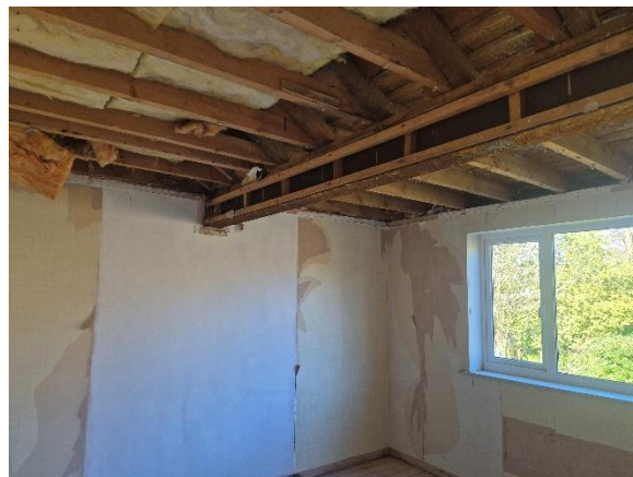
Photograph 12: Removed ceilings within B1.
