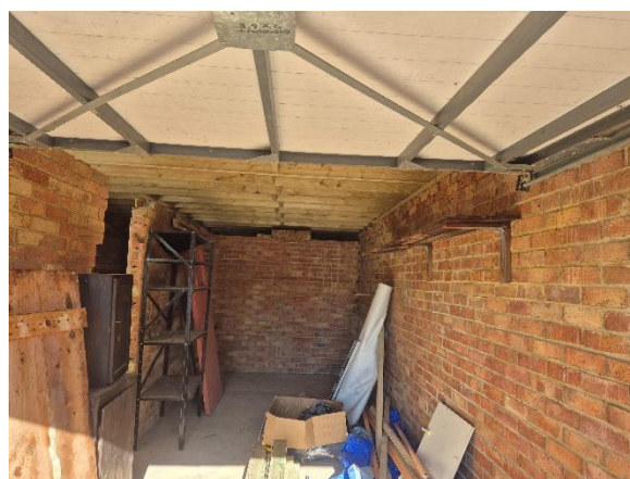
Photograph 16: Interior of the garage.
