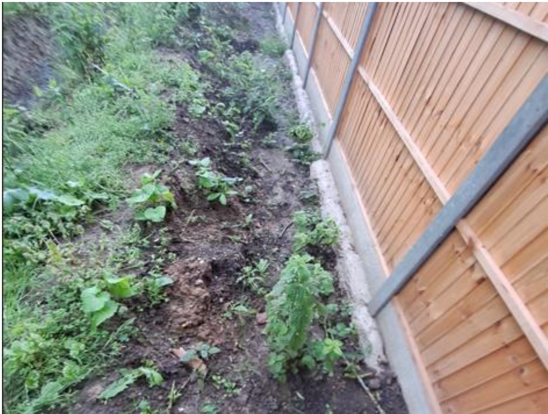
Fig. 4 – Concrete laid on existing soil level directly under fence kickboard
