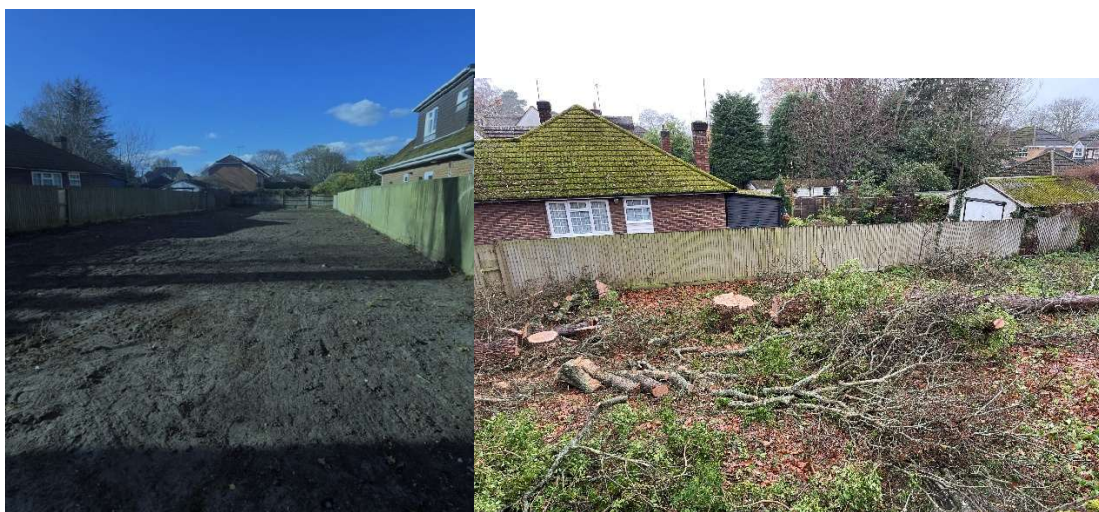
Site cleared since December 2024 and Trees including veteran tree cut down December 2024
