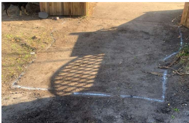
Area of tarmac shown at entrance
