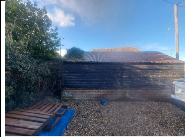
Photo 5: Garage, east elevation
