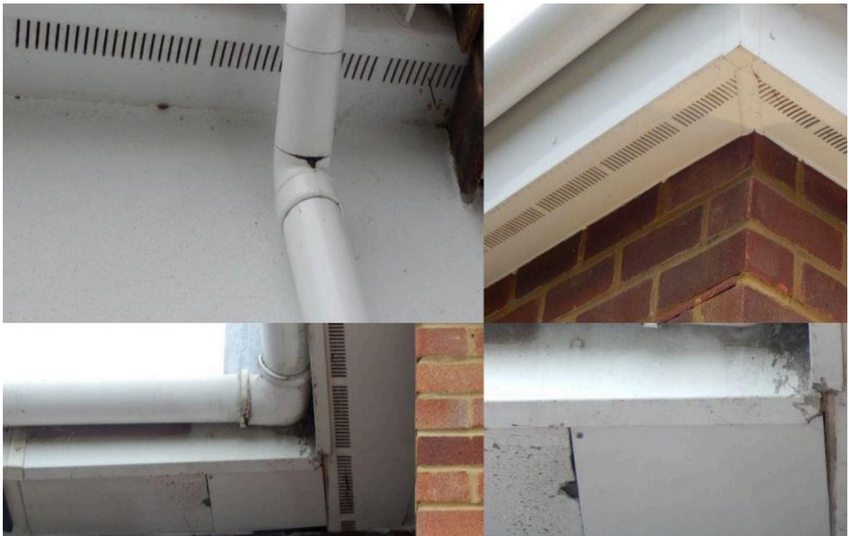
Image 6 – Close view of eaves coverings
