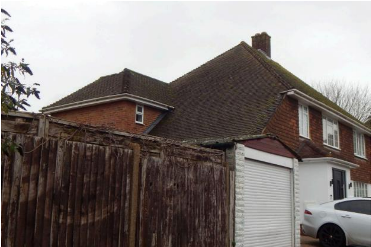
Image 3 – South facing elevation of the property
