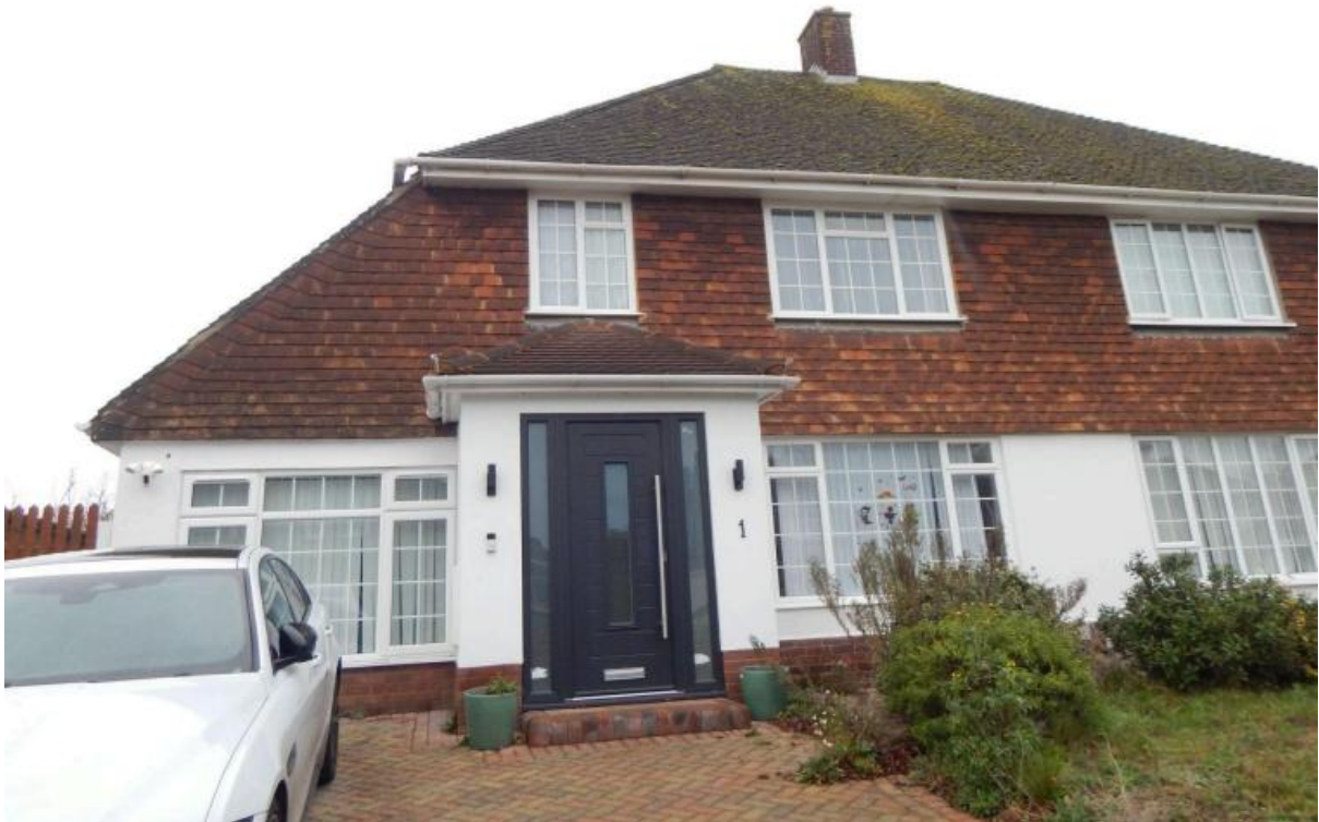
Image 1 – East facing elevation of the property
