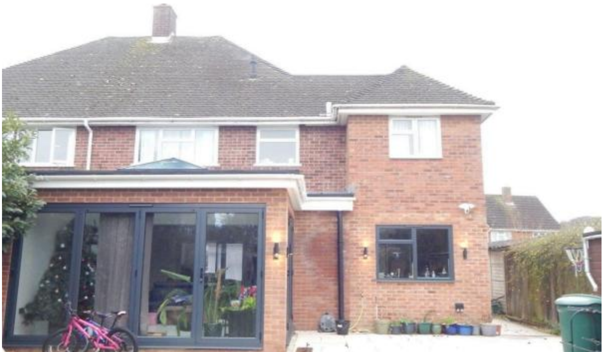
Image 2 – West facing elevation of the property
