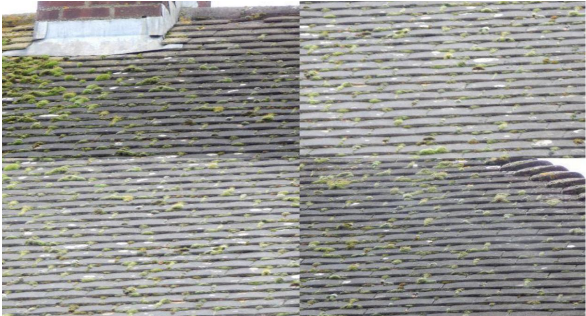
Image 5 – Example image of main tiled roof coverings to demonstrate condition throughout
