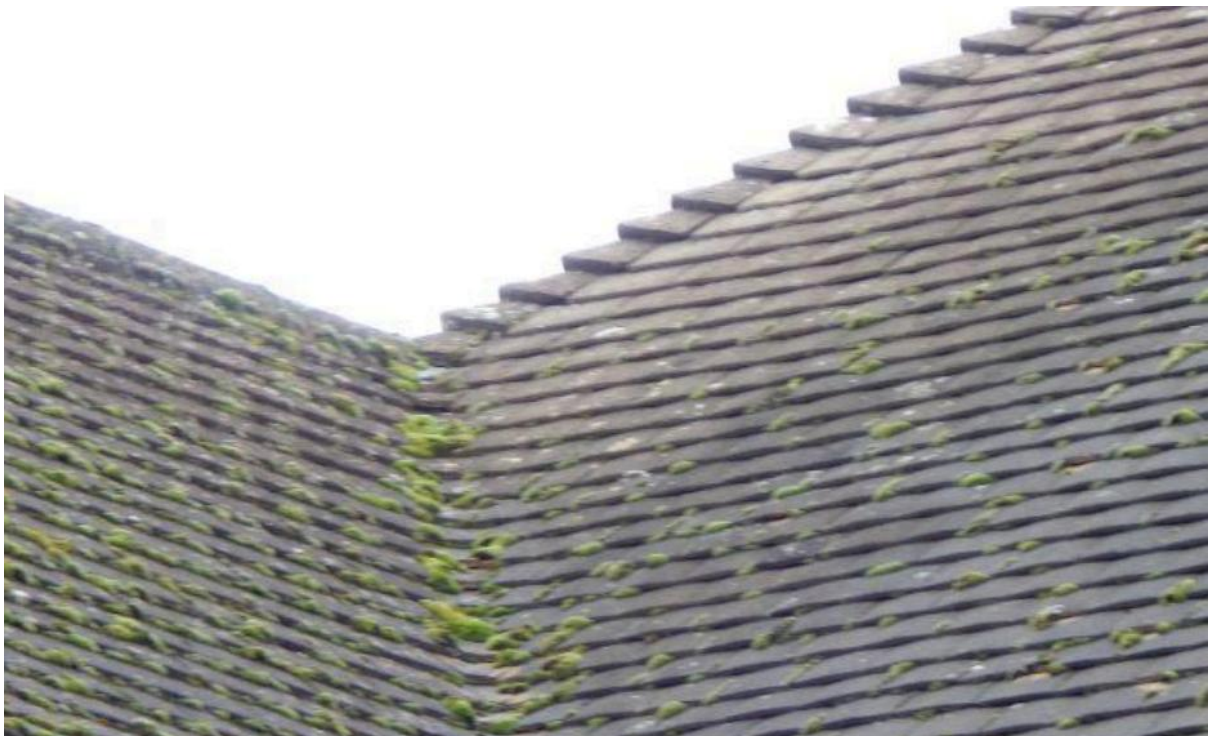
Image 4 – Example image of main tiled roof coverings to demonstrate condition throughout
