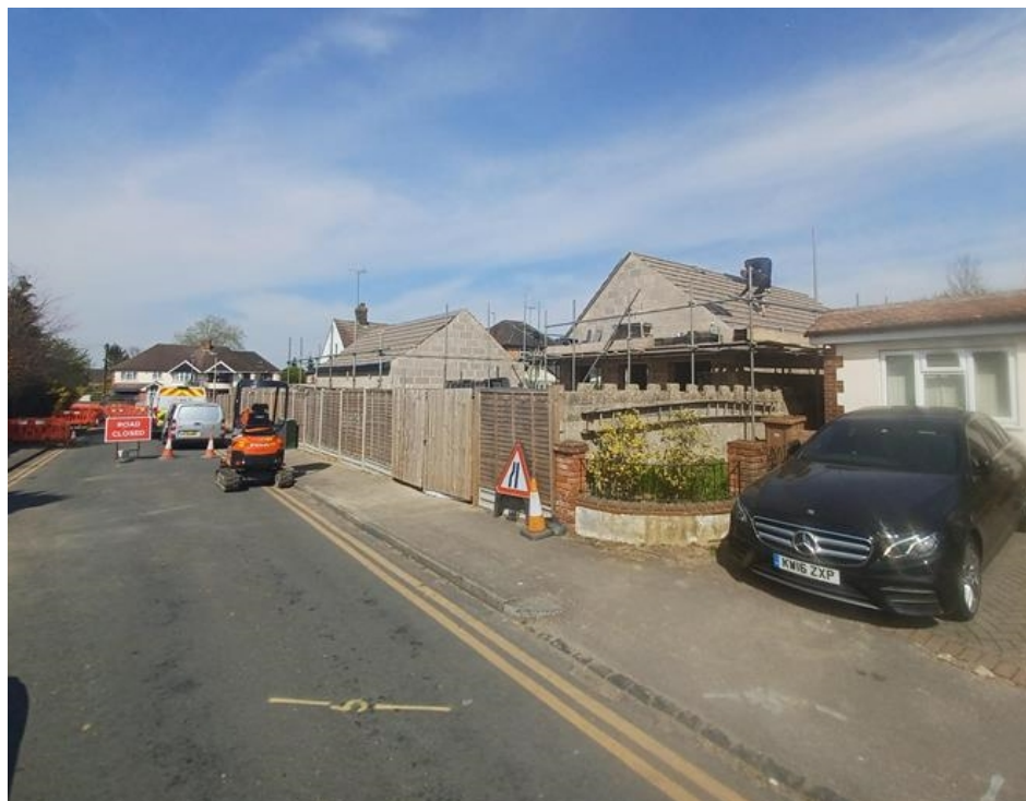
Figure 3 – Photograph taken in April 2025 showing the rear and south-western side boundary of the application site.
