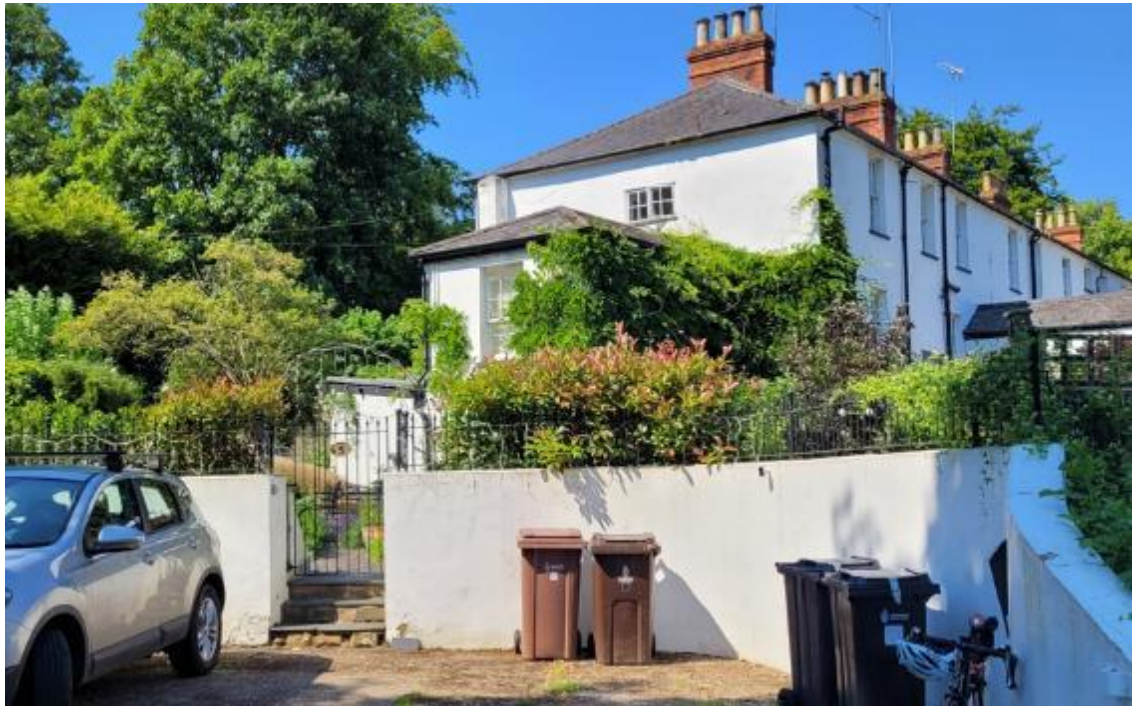
Property as viewed from Aston Lane
