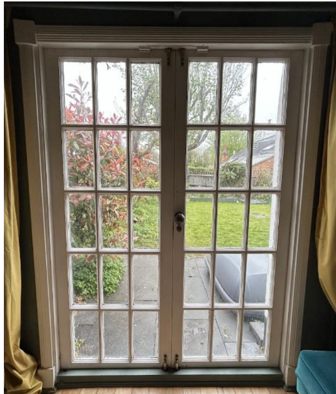
The existing internal architrave (pictured above) will be retained.
