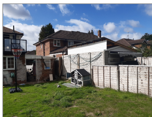
Figure 5 Image shows outbuilding at the rear of 31 Stanton Close that overshadows the rear habitable windows on the ground floor.
