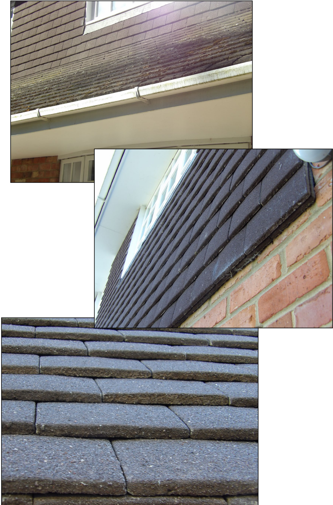
Figure 7. Example sealed cement hanging tiles on front and rear elevations. Orchard Cottage, Hurst. 18.03.25
