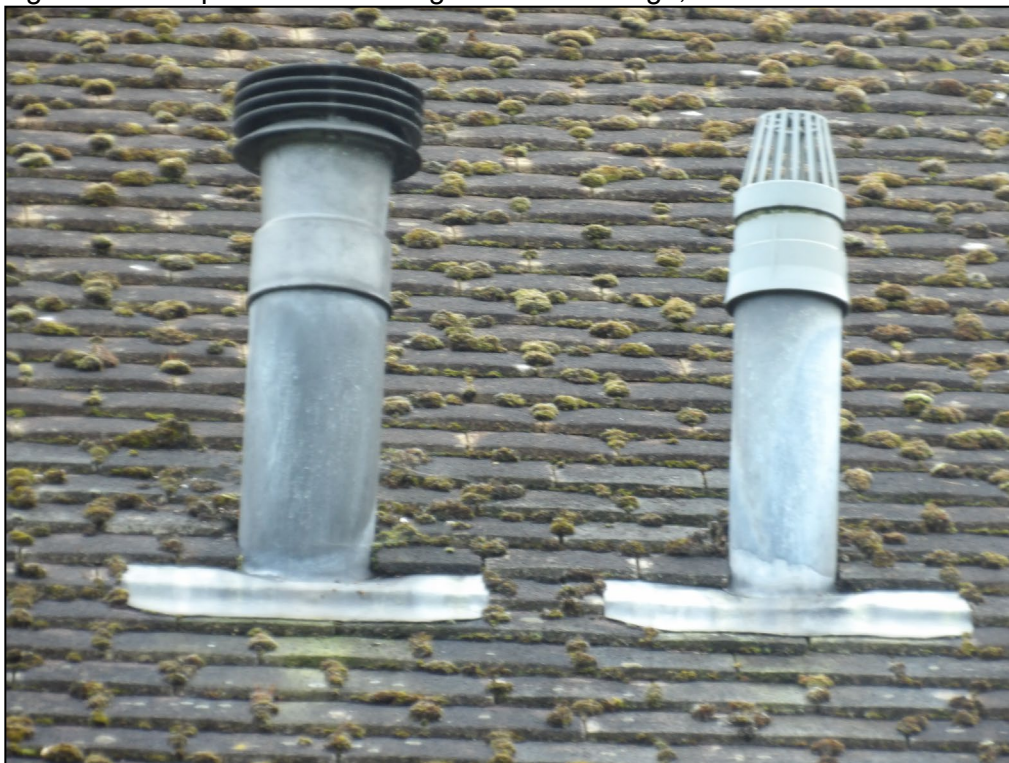
Figure 6. Example of lead flashing. Orchard Cottage, Hurst. 18.03.25
