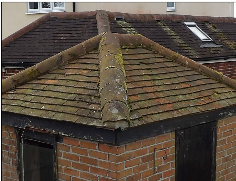
Figure 12. Rear view of moved tiles and rotten fascia on outbuilding. 5 Walden Avenue, Arborfield. 25.02.25
