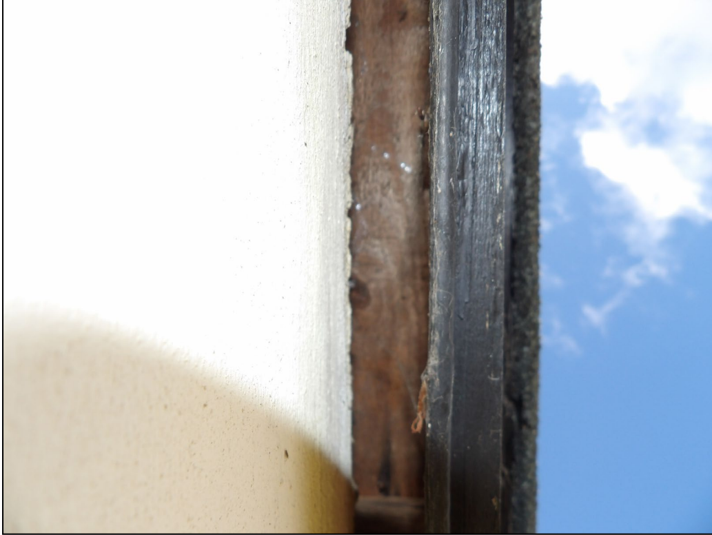
Figure 8. Example gap between fascia and wall plate on rear extensions. 5 Walden Avenue, Arborfield. 25.02.25
