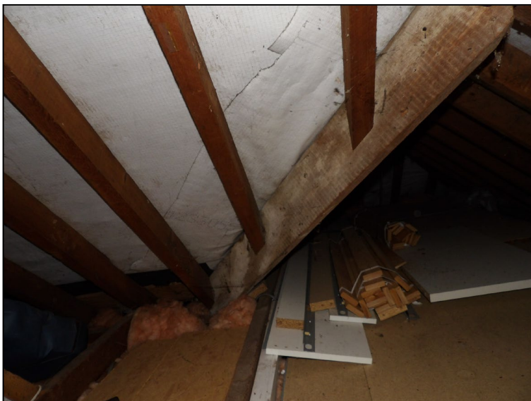
Figure 14. Membrane lining to tiles in eaves storage areas. 5 Walden Avenue, Arborfield. 25.02.25
