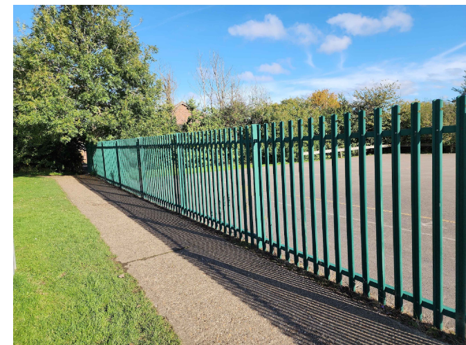
Existing Palisade Fencing
