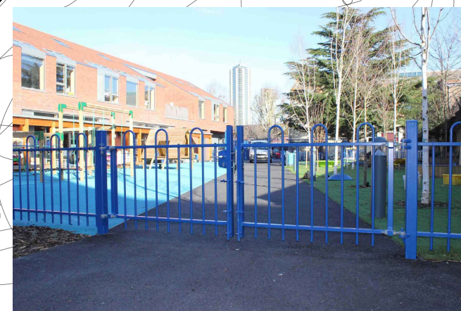
Low Level Fencing
