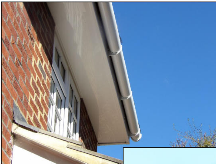
Figure 11. Example of sealed soffit and fascias. 8 Braybrooke Gardens, Wargrave. 16.09.25
