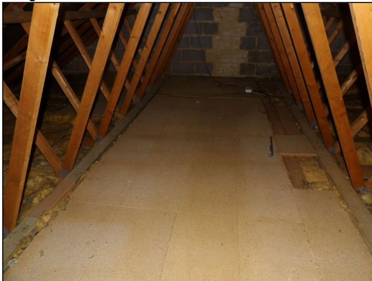
Figure 12. Example main loft space and bitumen lining to tiles. 8 Braybrooke Gardens, Wargrave. 16.09.25
