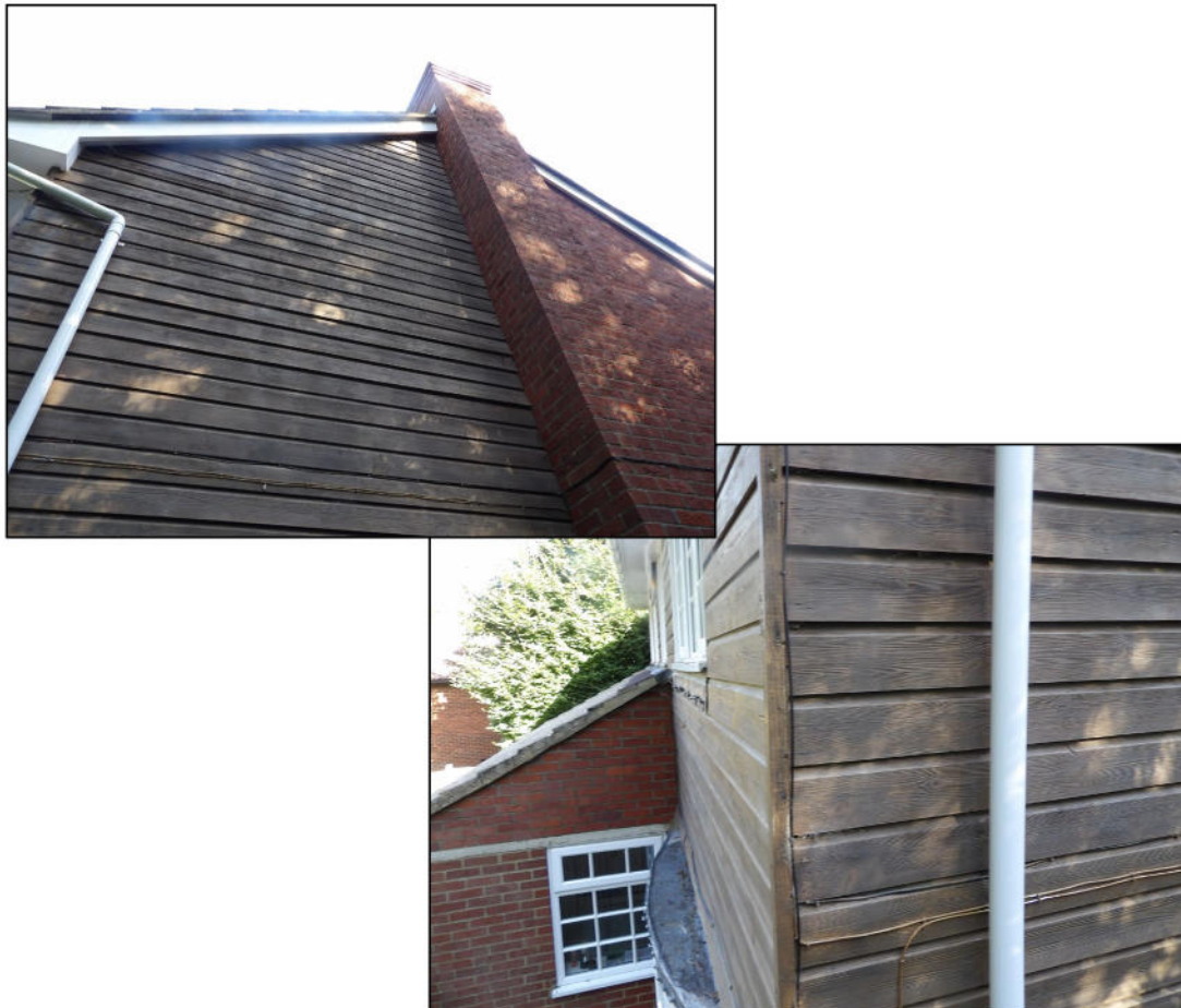
Figure 7. Example of tightly fitted wooden cladding. 8 Braybrooke Gardens, Wargrave. 16.09.25
