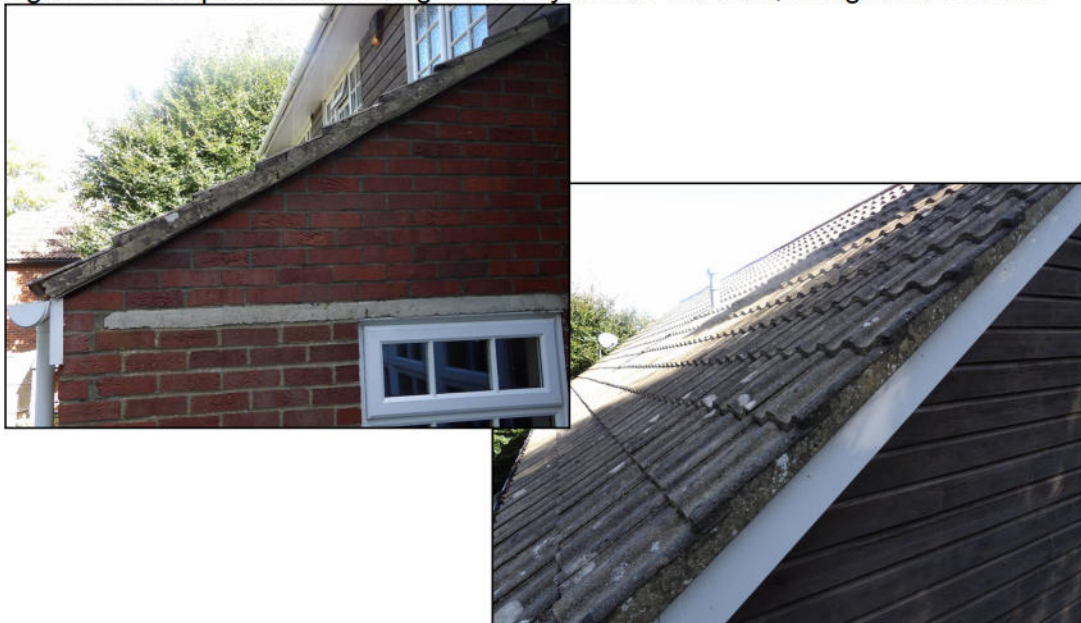
Figure 5. Example of sealed verges. 8 Braybrooke Gardens, Wargrave. 16.09.25
