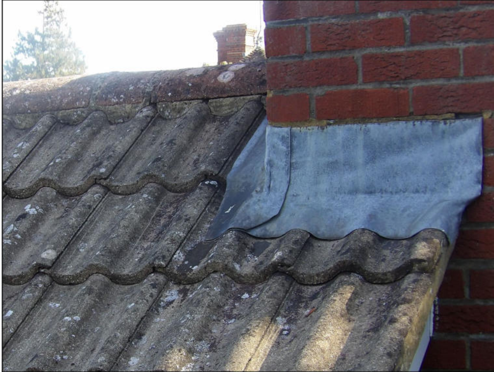
Figure 6. Example sealed lead flashing around the chimney stack. 8 Braybrooke Gardens, Wargrave. 16.09.25
