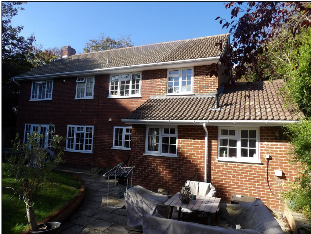
Figure 9. Rear view of property and historical extensions. 8 Braybrooke Gardens, Wargrave. 16.09.25
