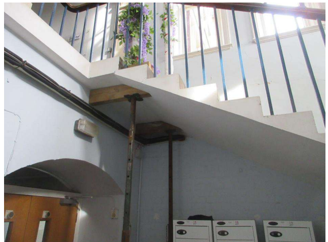
Figure 3. Back propping beneath the ground floor landing to transfer loads to ground level.
