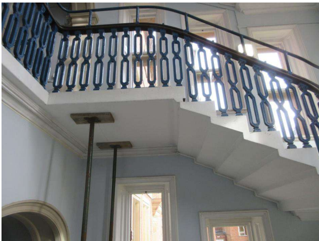
Figure 2. Acrow props supporting the first-floor landing from below.
