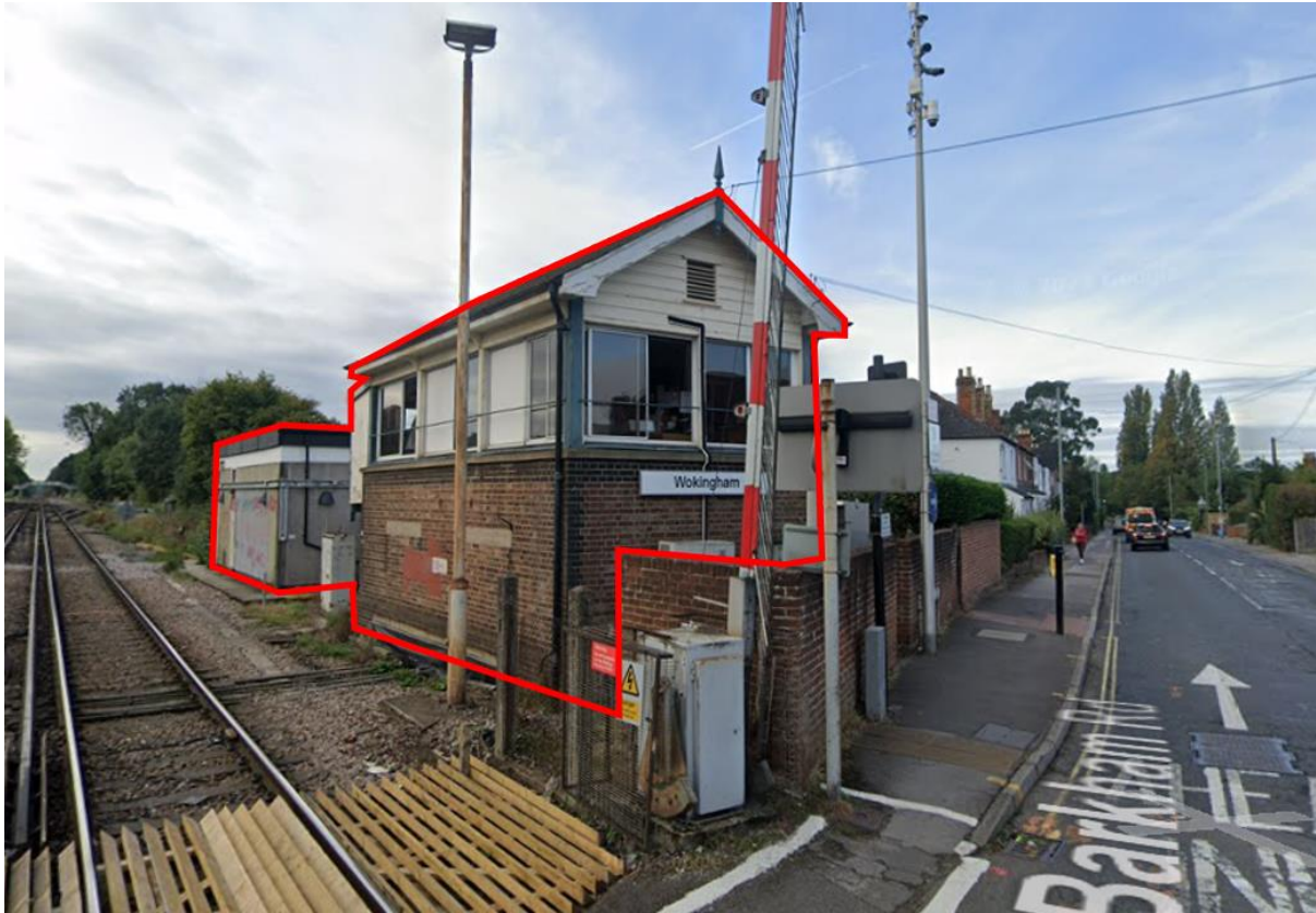
Figure 1 - Photograph of signal box and operational equipment building from Barkham Road (buildings to be demolished edged in red) (Google, 2025)
