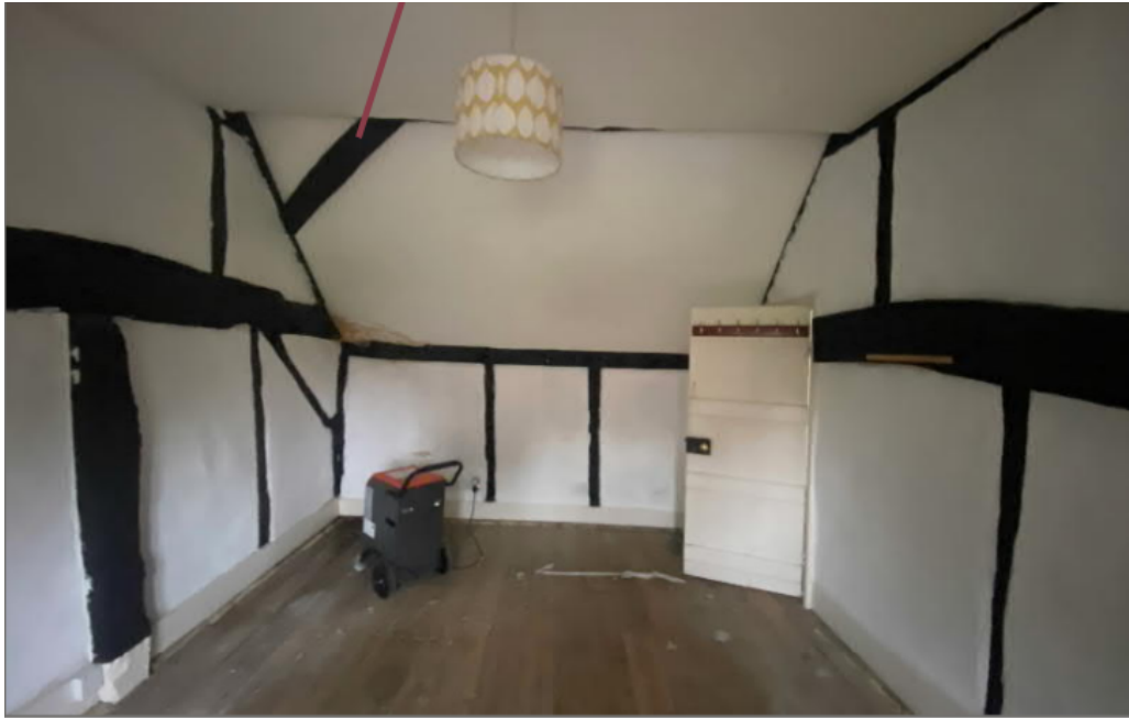
LHS of the first floor front room looking towards back wall of lateC16th cottage– with the C20 th extension behind.
