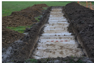
Plate 1: Mitigation Trench 35 view to South. 1m scale.
