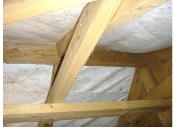
10. Breathable roofing membrane lining roof (B1).
