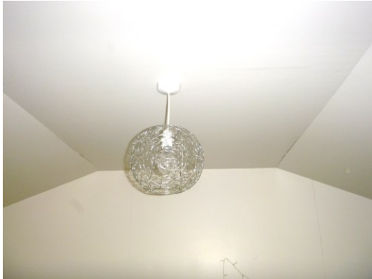
12. Walls and ceiling plastered in summerhouse (B2).
