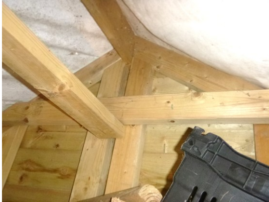
11. Single-skin shed panel walls with tight roof timbers at gable ends (B1).
