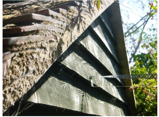
6. Intact verge mortar on northern gable (B1).
