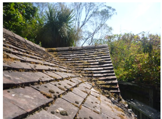
2. Mostly flat and tight overlapping roof tiles (B1).
