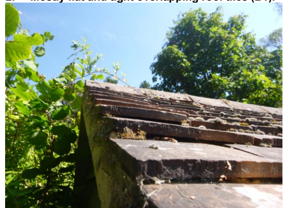
4. Inspected gaps under slightly raised verge tiles at eastern gable end (B1).
