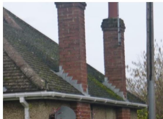
Photograph 6. Lead flashing sealed to brickwork and roof tiles (southeast elevation).
