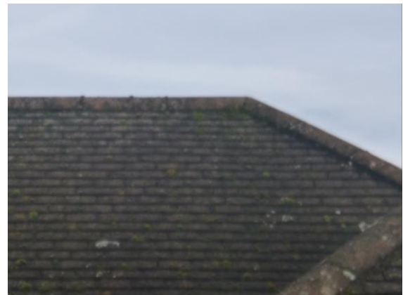
Photograph 4. Ridge and hip mortar fully intact (front elevation).
