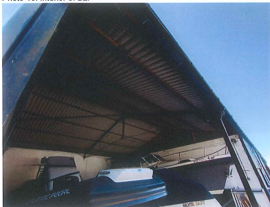
Photo 10: Interior of B2.
