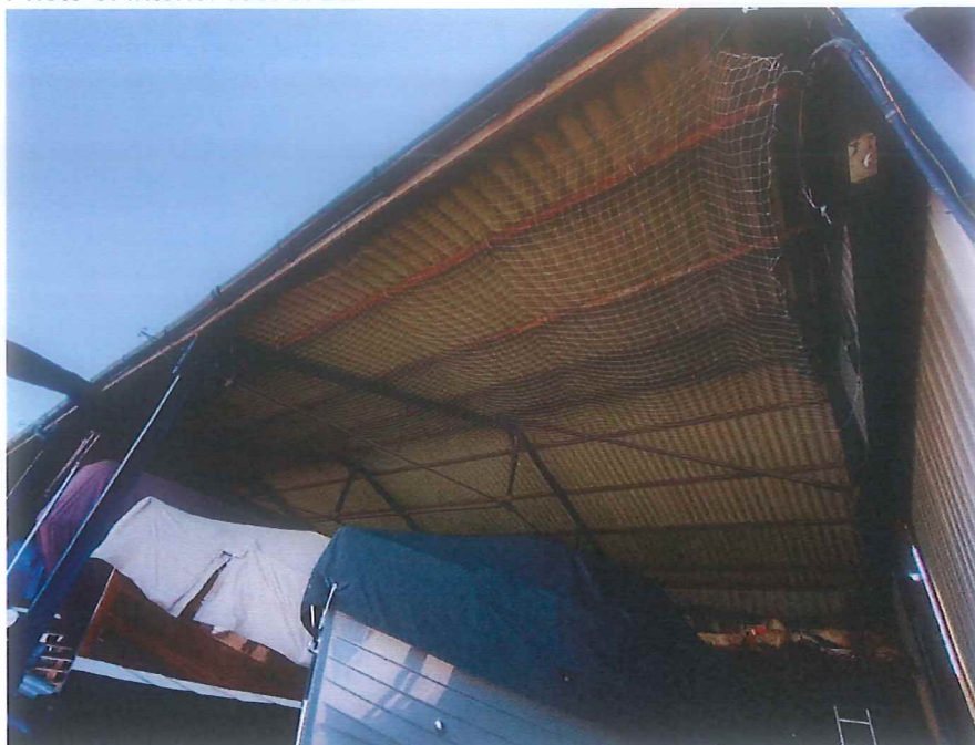
Photo 9: Interior roof of B2.
