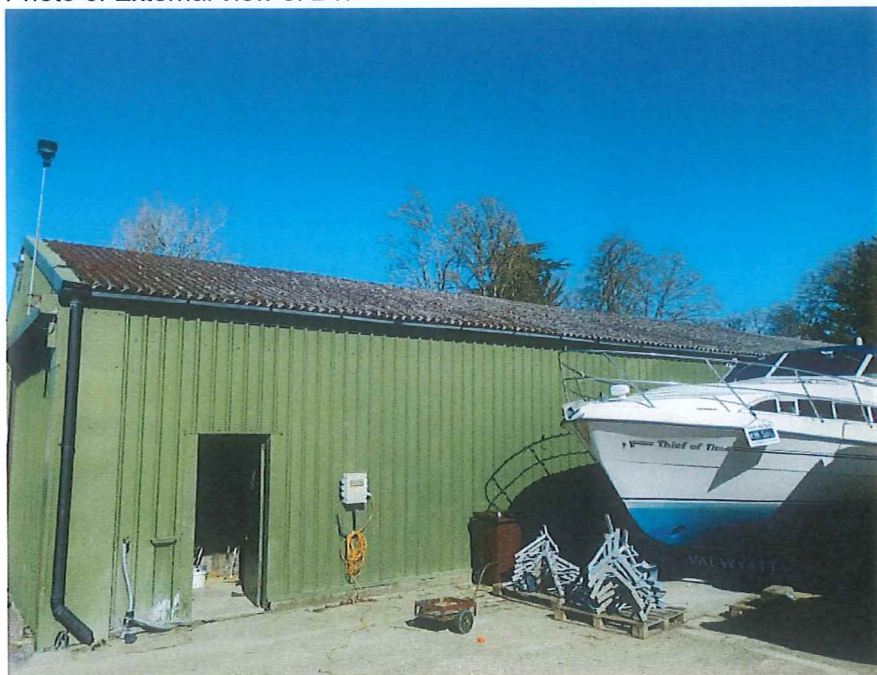
Photo 8: External view of B1.
