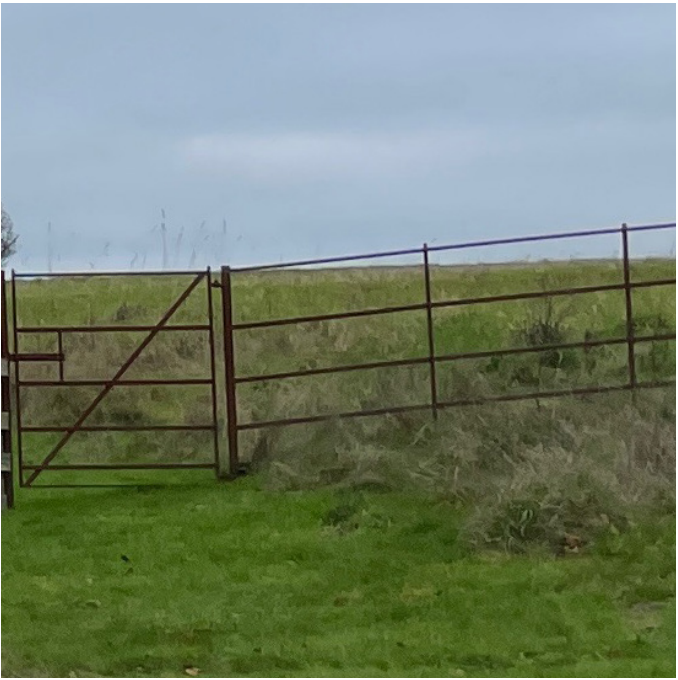
B06 (Q40/521) Single field gate Supplier: Britannia metalwork. Material: Wrought iron, weathered finish
