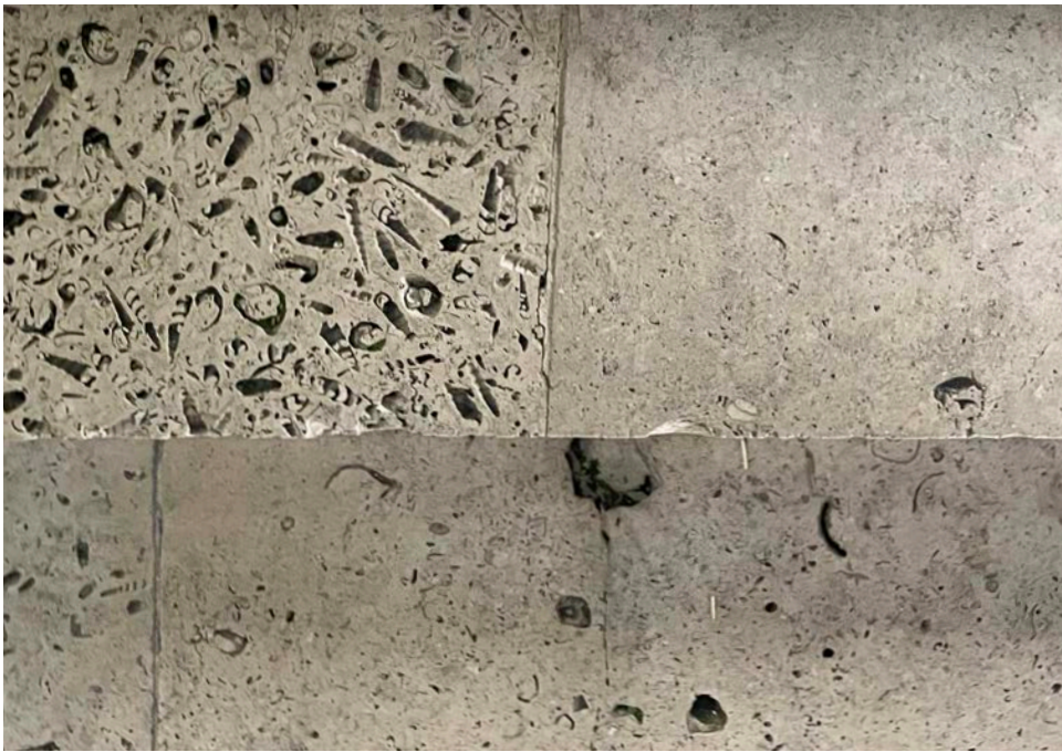
P01 (Q25/110) & P04 (L37/110) Portland stone paving and steps
