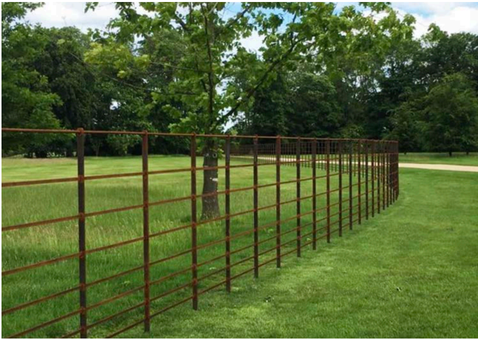
B01 (Q40/371) Deer-proof fencing Height: 1800mm Supplier: Britannia metalwork. Material: Wrought iron, weathered finish
