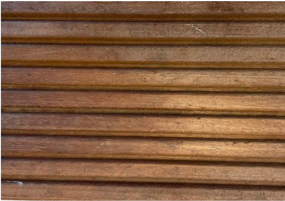
P07A/B (Q55) Pontoon and Deck FSC thermo iroko, 1400 x 38mm boards, with 200 mm posts
