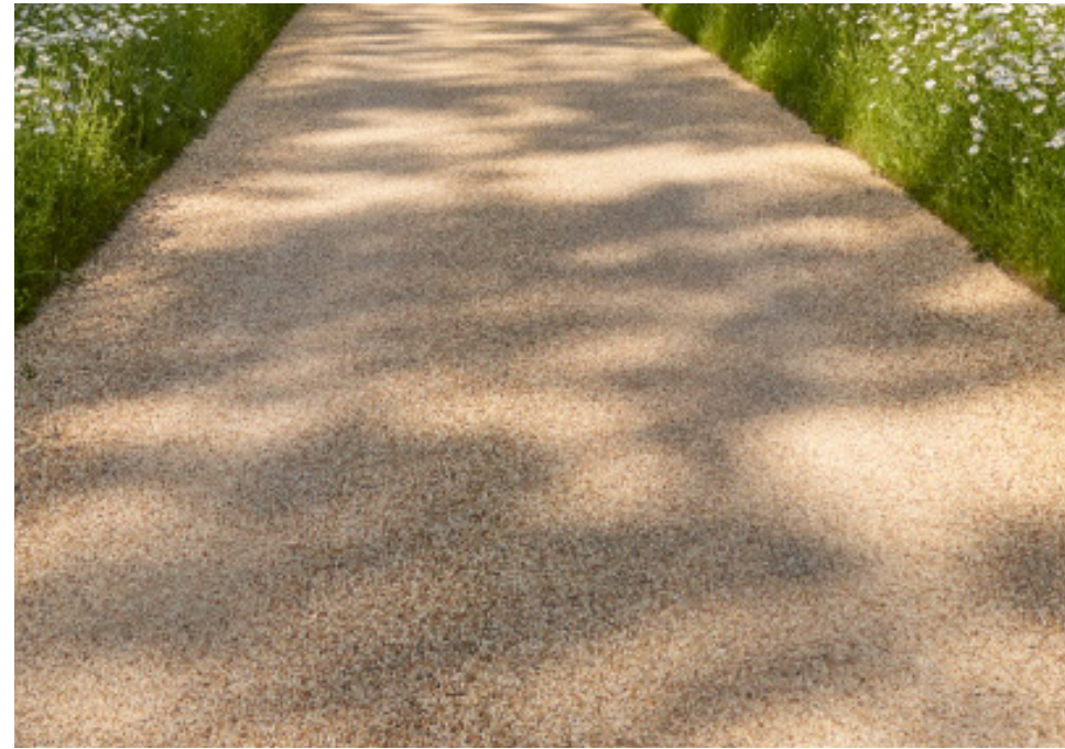
P06 (Q22/110) Tar and Chip Coated chippings
