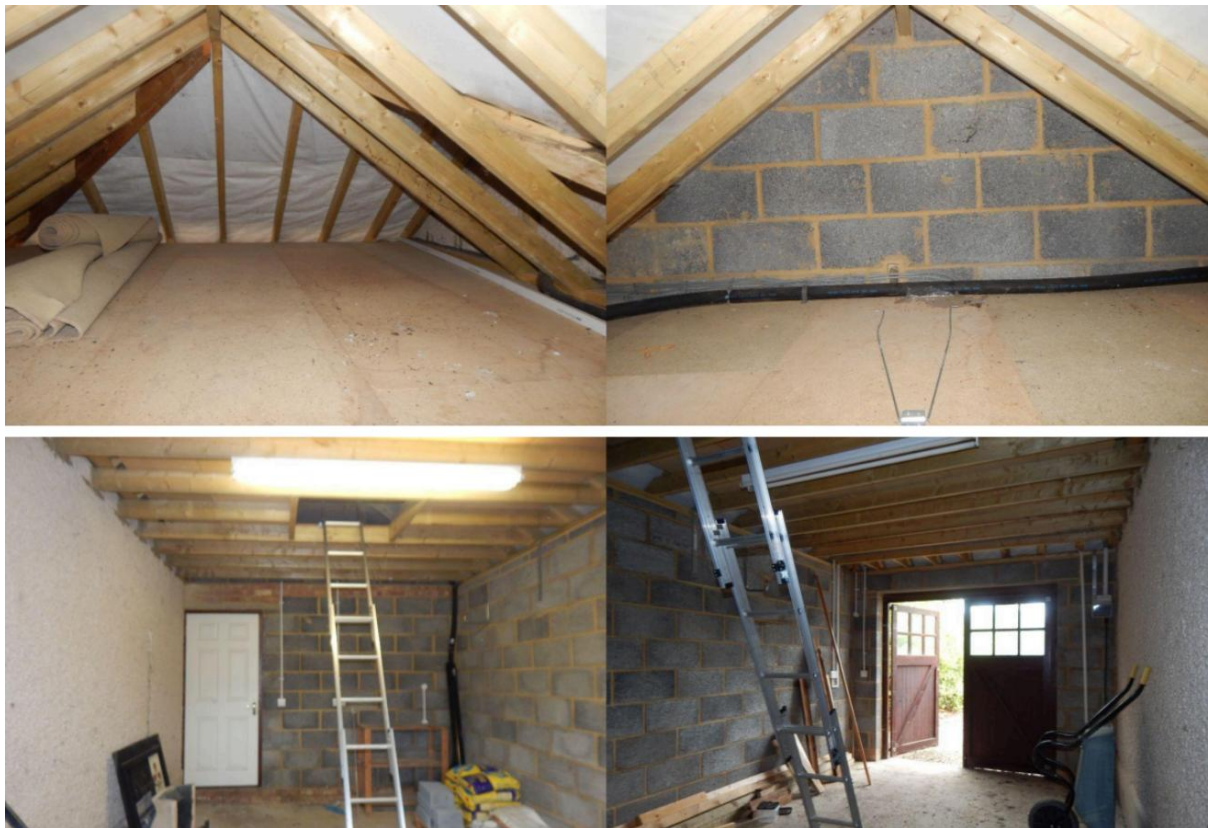
Image 11 – Internal views from within the garage section of the property
