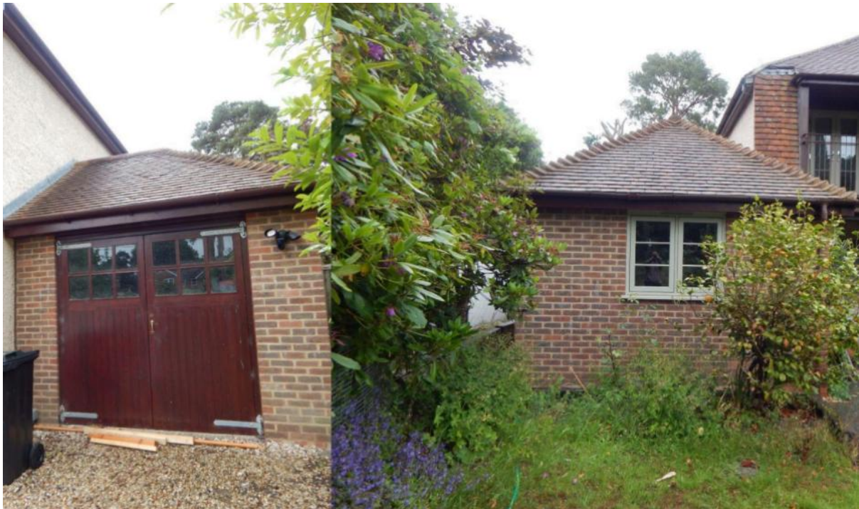
Image 9 – North & South facing elevation of the linked garage which is situated across the West elevation of the property
