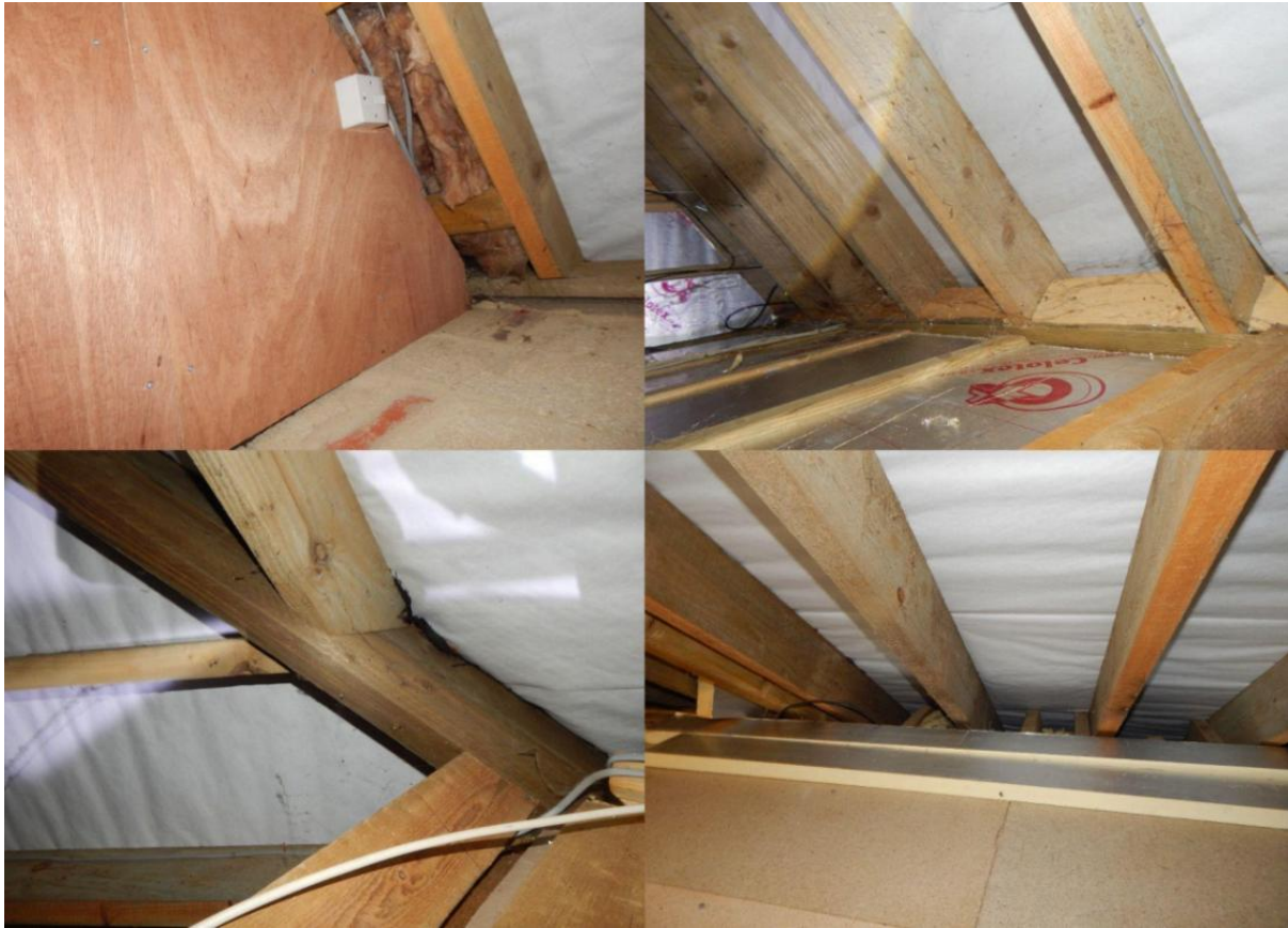
Image 13 – Internal views from within the accessible roof void spaces of the property
