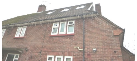
Photograph 5. Ridge, hip and verge mortar fully intact (front elevation).
