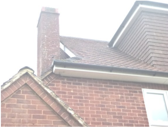
Photograph 8. uPVC soffit sealed to brickwork walls (rear elevation).
