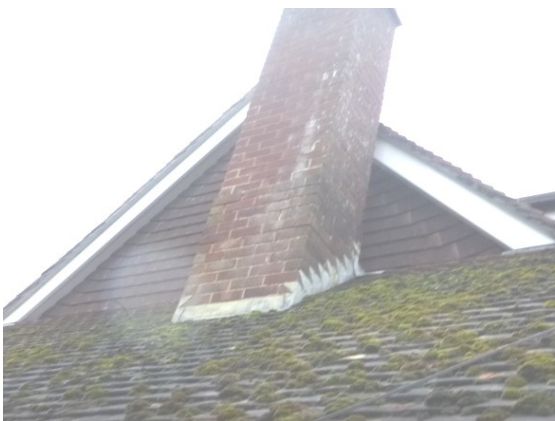
Photograph 6. Sealed lead flashing and hanging tiles (north elevation).
