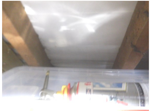
Photograph 10. Fully intact breathable roofing membrane (Eaves Space 2).
