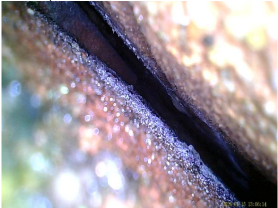
Photograph 4. Endoscope check of lifted tiles at the existing extension.
