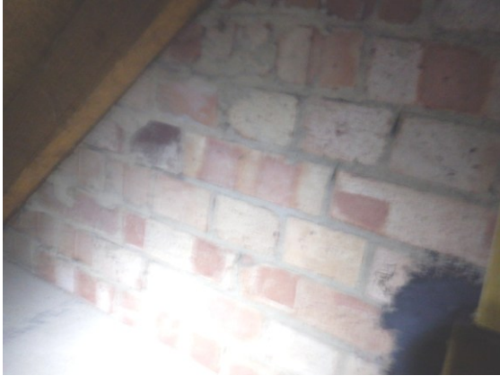
Photograph 11. Timbers sealed to brickwork gable (Eaves Space 1).
