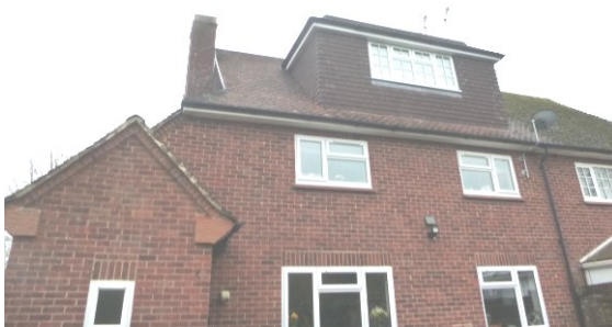
Photograph 1. Rear of property viewed from west.
