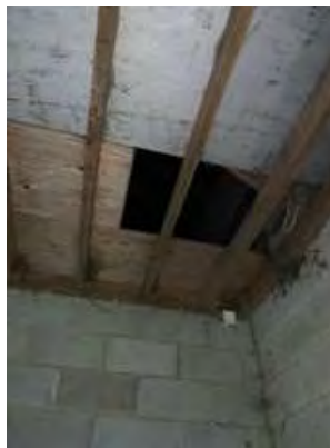
Photo 71 Building B3 – loft hatch used by BLE
