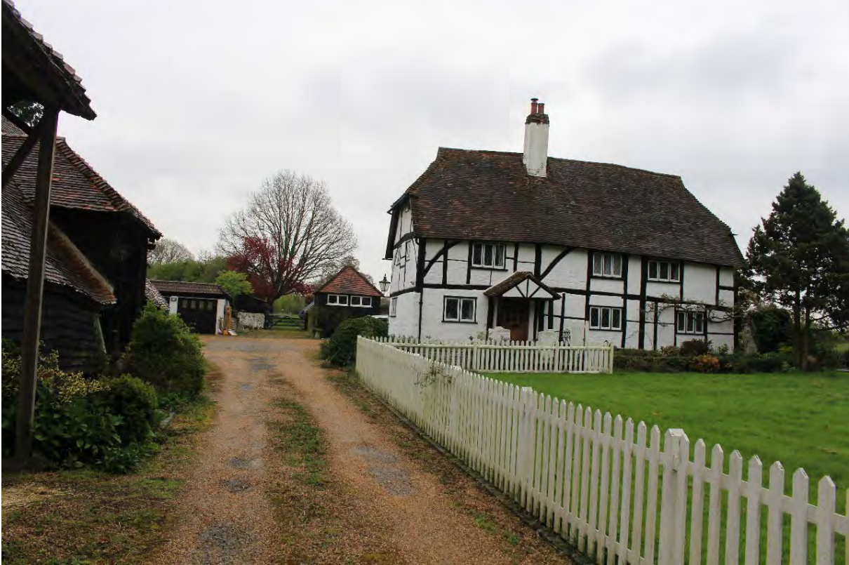
Image EDP A1.1: West facing view of Pearce's Farmhouse ( 1319115 ) and granary ( 1135768 ) from the driveway entrance to Pearce's Farm along Easthampstead Road. The farmhouse's traditional 15 th -17 th century vernacular architectural style is shown alongside the view from the driveway approach to the farmhouse.
