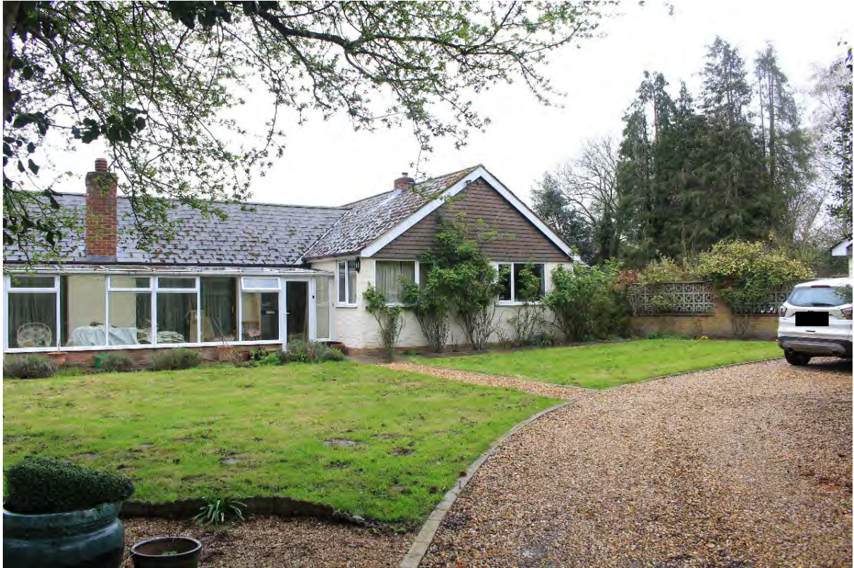
Image EDP A1.7: North facing view from the driveway to Pearce's Farm. View of the post-1970s modern cottage building, illustrating an unsympathetic design and use of modern materials, not in keeping with the character of Pearce's Farmhouse ( 1319115 ) or its associated barn ( 1118118 ) located opposite the modern cottage.
