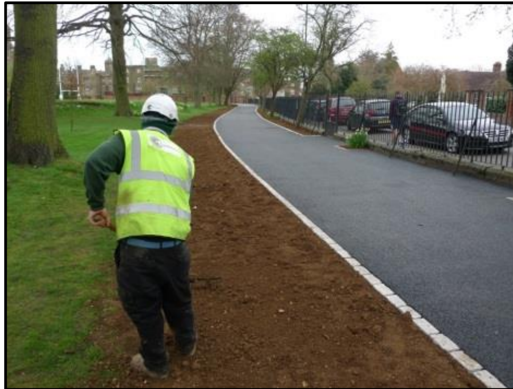
Fig 17 – In the event of 'making good' topsoil will be BS3882 compliant and raked out by hand to no greater depth than 100mm.
