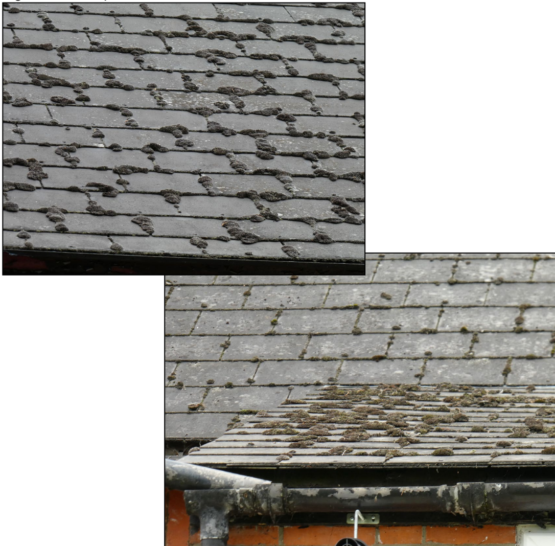
Figure 4. Example of roof tiles. 1 Diamond Villas, Hurst. 10.09.24
