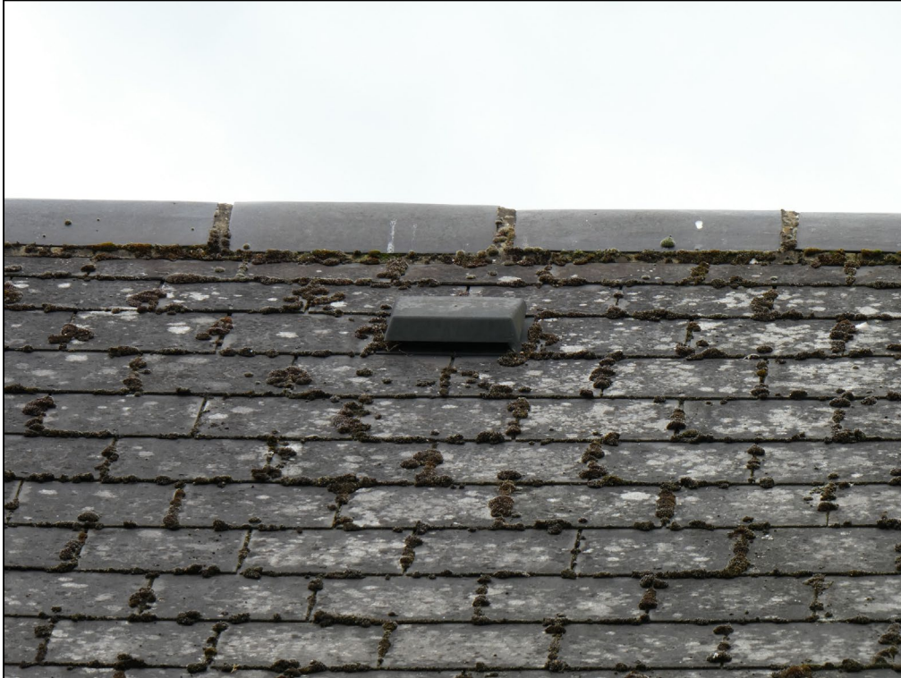
Figure 5. Example of ridge tiles. 1 Diamond Villas, Hurst. 10.09.24
