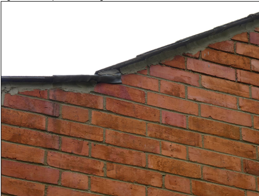
Figure 6. Example sealed verges. 1 Diamond Villas, Hurst. 10.09.24
