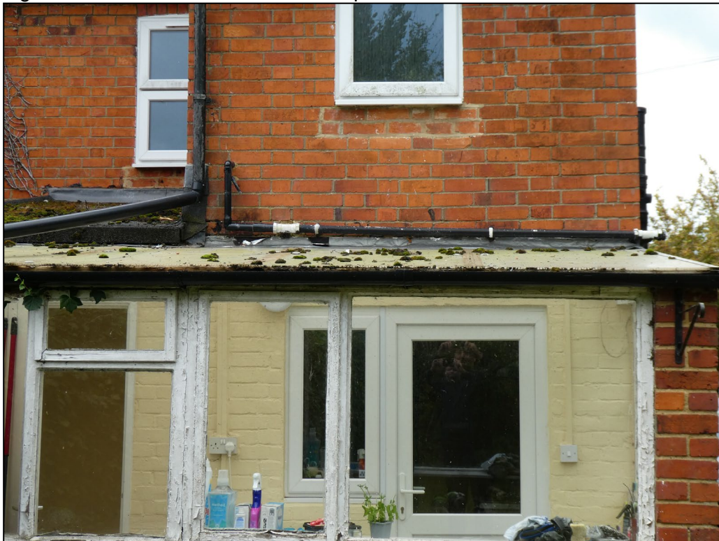
Figure 8. Rear summer room and Perspex roof. 1 Diamond Villas, Hurst. 10.09.24
