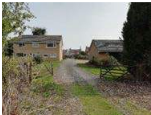
Photo looking east showing the access point to the site, via the residential property with associated garage.
