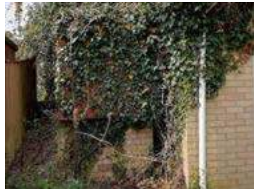
Photo looking west showing above ground fuel storage tank next to the single storey brick garage located to the adjacent south of the route of the proposed access road.
